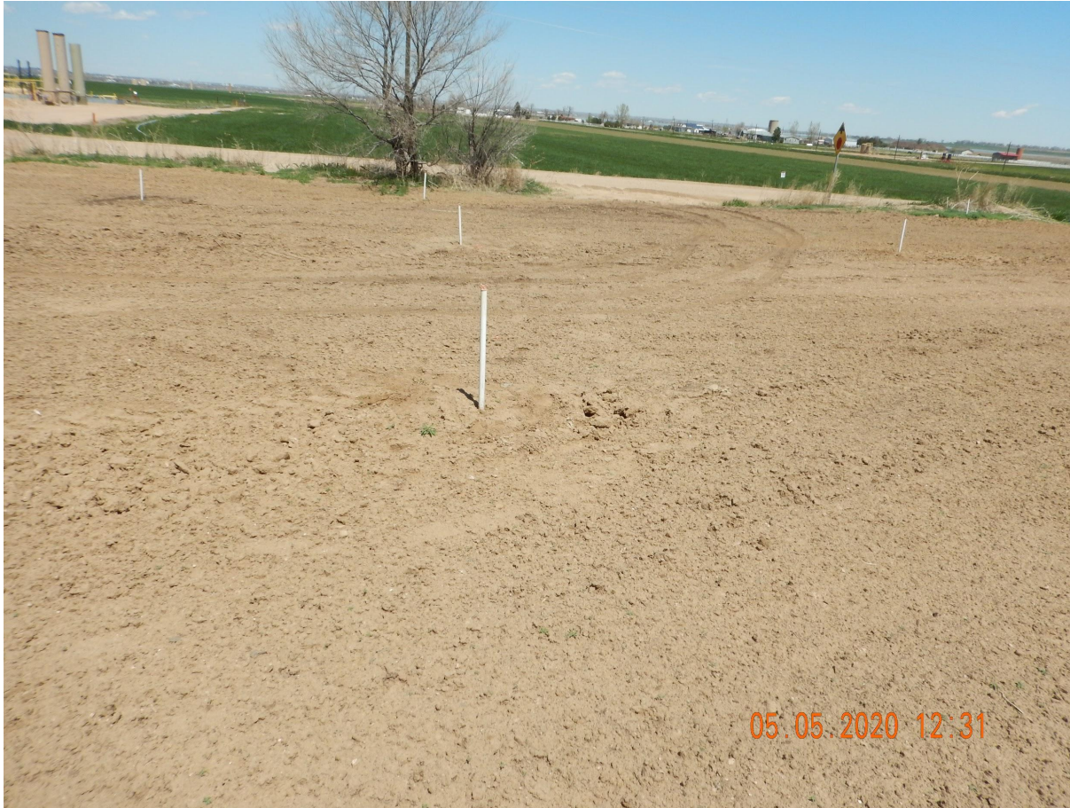
Photo 5. Photo taken from the associated offsite tank battery, facing North. Photo illustrates vehicle traffic. Operator should consider temporarily fencing off the area as this is not stabilized and to help promote successful vegetation establishment to stabilize the area.
