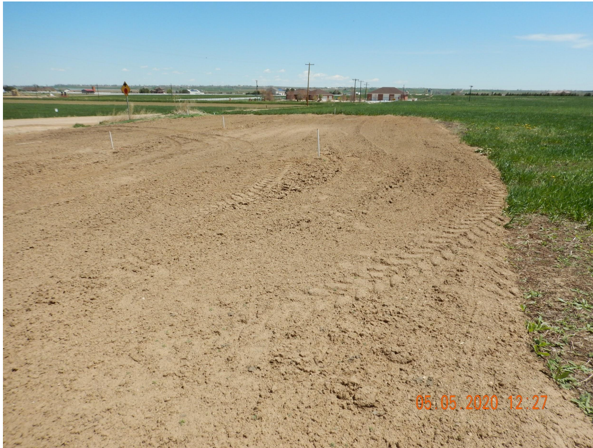
Photo 4. Photo taken from the associated offsite tank battery, facing East. Photo illustrates Operator has performed some of the final reclamation requirements (i.e., remove gravel). However, there was very little germination of desirable species; therefore, it does not appear the tank battery has been seeded. Also, there is an active remediation.
