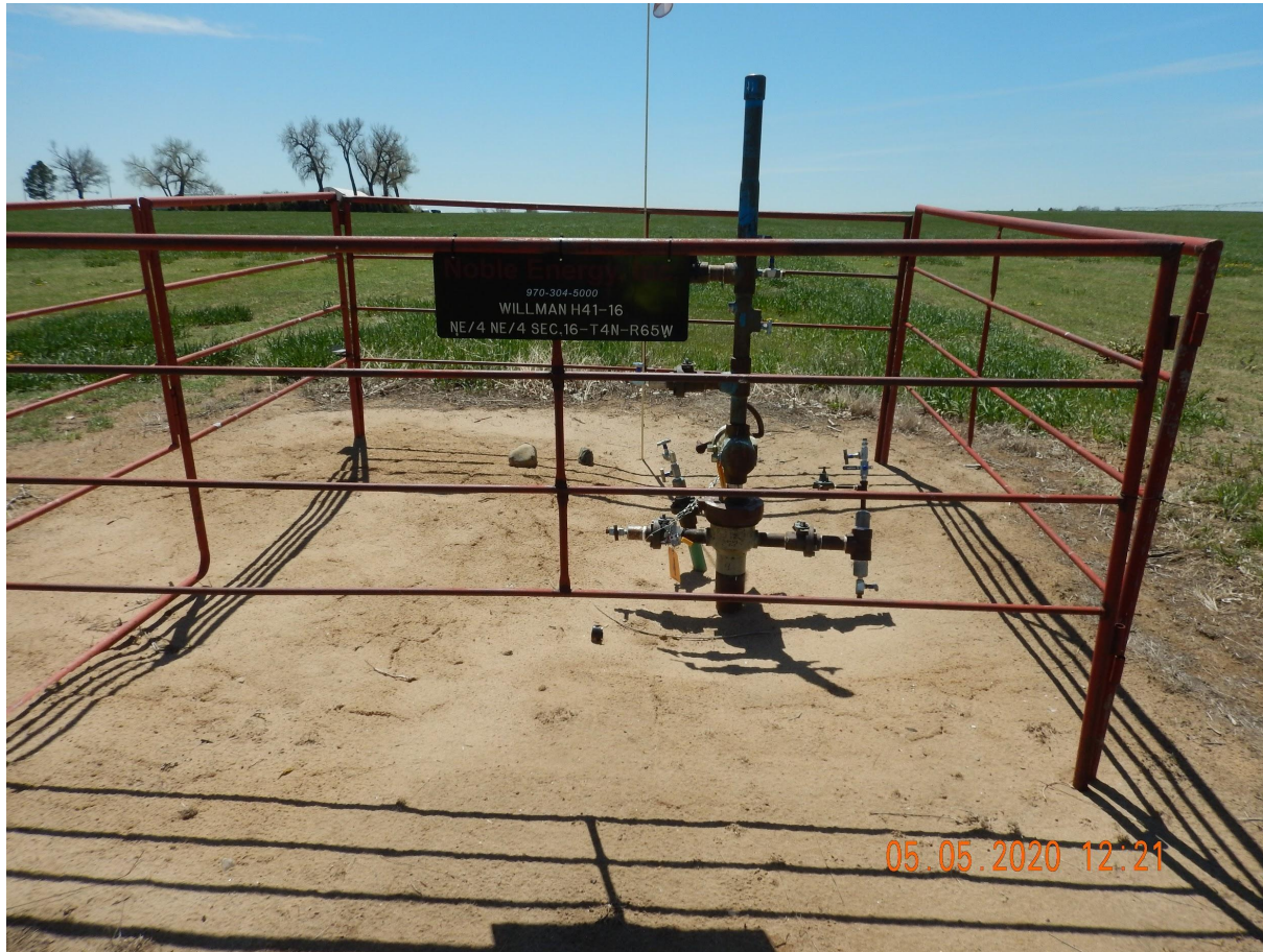
Photo 2. Photo taken of the TA well, facing South. Photo illustrates the TA well appears to be locked out and tagged per the variance.
