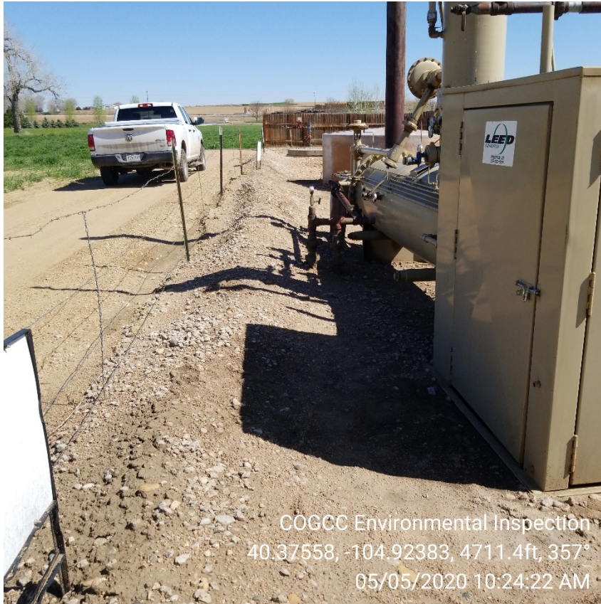
Photo 1 – Separator and fiberglass produced water vault.
