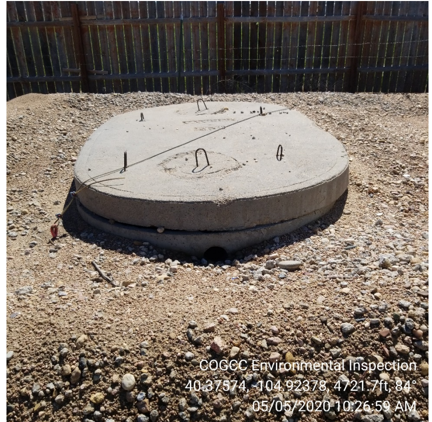
Photo 2 – Concrete produced water vault.
