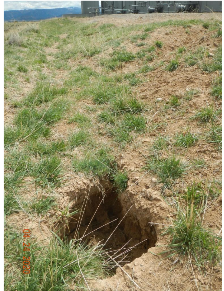
Photo#3: Sinkhole off ditch leading from pad.
