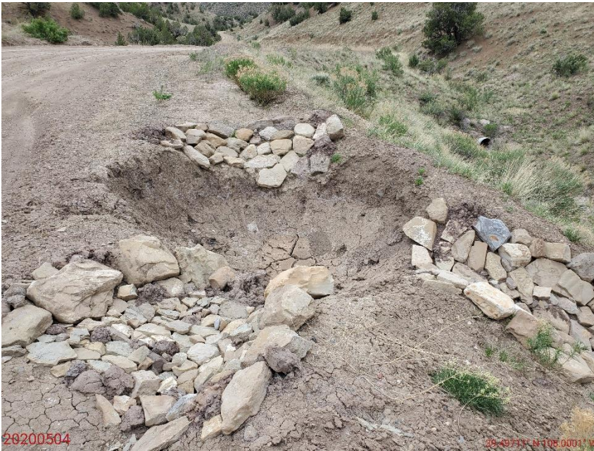
Photo 3: Photo taken from the west end of the Location, facing south. Photo shows sediment trap; Trap appears to have sufficient inlet/outlet armoring.
