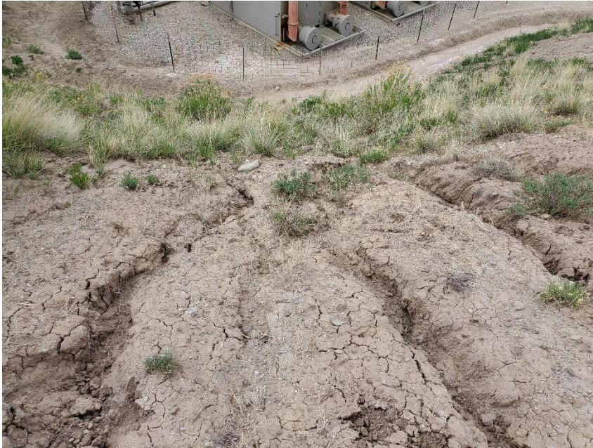
Photo 9: Photo taken from the slopes on the east end of the Location, facing west. Photo shows areas where Operator appears to have pushed soils upon a hillside of the Location. Photo shows slopes have not been stabilized and erosion degradation is evident
