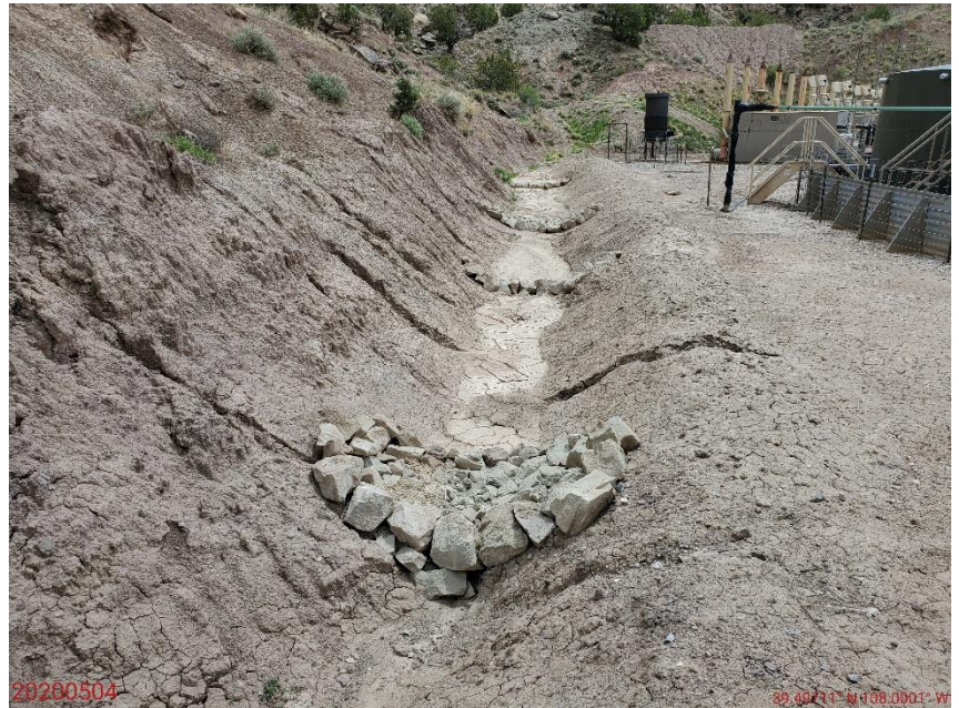
Photo 6: Photo taken from the stormwater diversion ditch on the northeast end of the Location. Photo shows velocity checks within ditch appear to be in proper functioning condition. Erosion degradation along areas of the ditch evident; Sediment deposition with ditch (advise maintenance).
