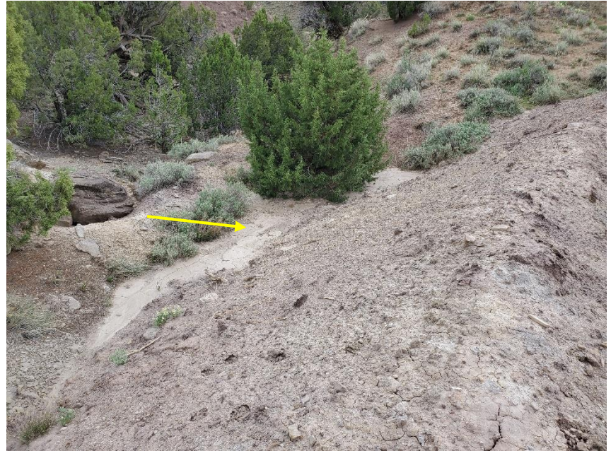
Photo 10: Photo taken from the slopes on the east end of the Location, facing east. Photo shows areas where Operator appears to have pushed soils upon a hillside of the Location. Photo shows missing or insufficient BMPs in places on the eastern end of the soils to prevent sediment transport off location into another drainage; Photo also shows sediment deposition off Location.
