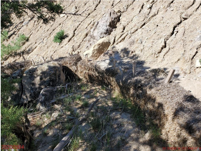
Photo 15: Photo taken from the southeast end of the Location/Location entrance, facing south. Photo shows sediment has filled areas between the slope and the erosion bales. BMP is no longer in proper functioning condition.
