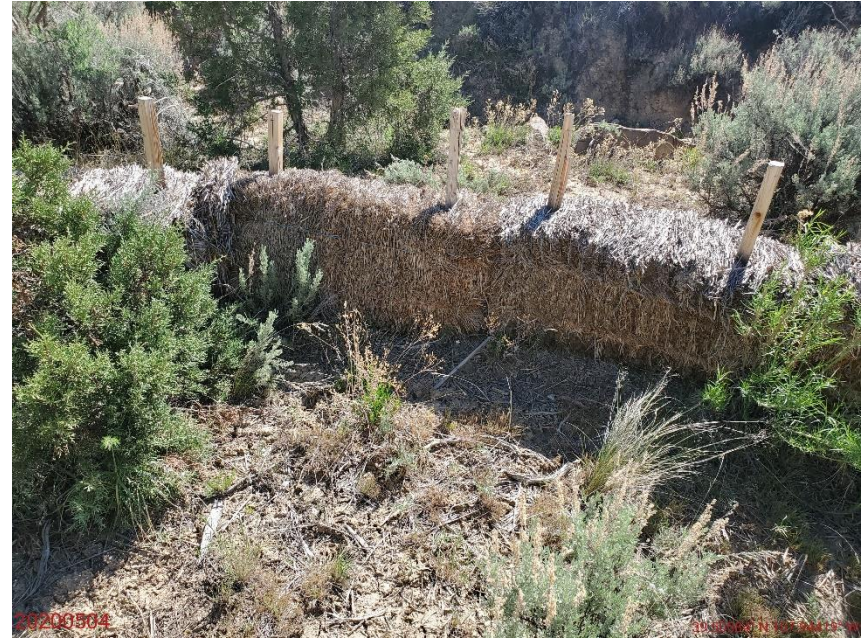
Photo 14: Photo of erosion bales on the eastern perimeter of the Location. Erosion bales are temporary sediment control structures that are required to be entrenched. Photo shows BMP has not been entrenched; BMP has not been installed in accordance with good engineering practices.
