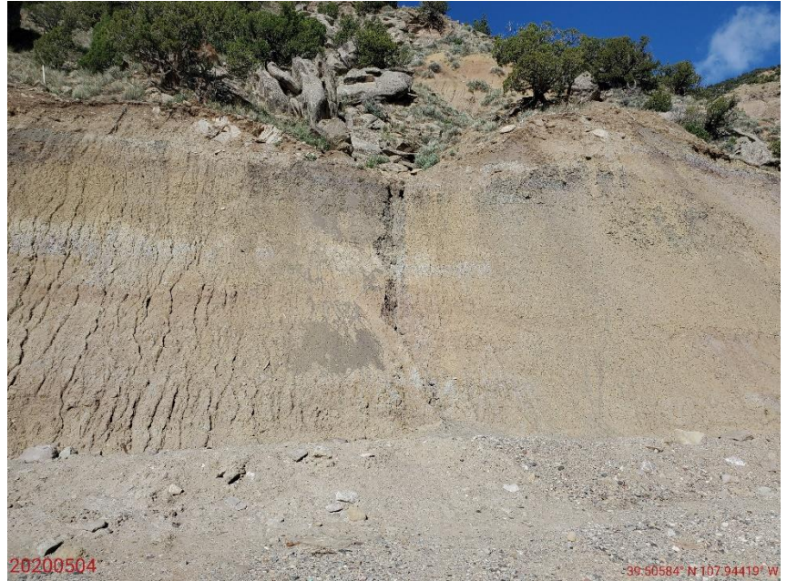
Photo 6: Photo taken from the west end of the Location, facing west. Photo shows erosion degradation on the cut slopes; Insufficient BMPs, or BMPs missing, to stabilize the slopes, manage runoff and prevent degradation to the Location.
