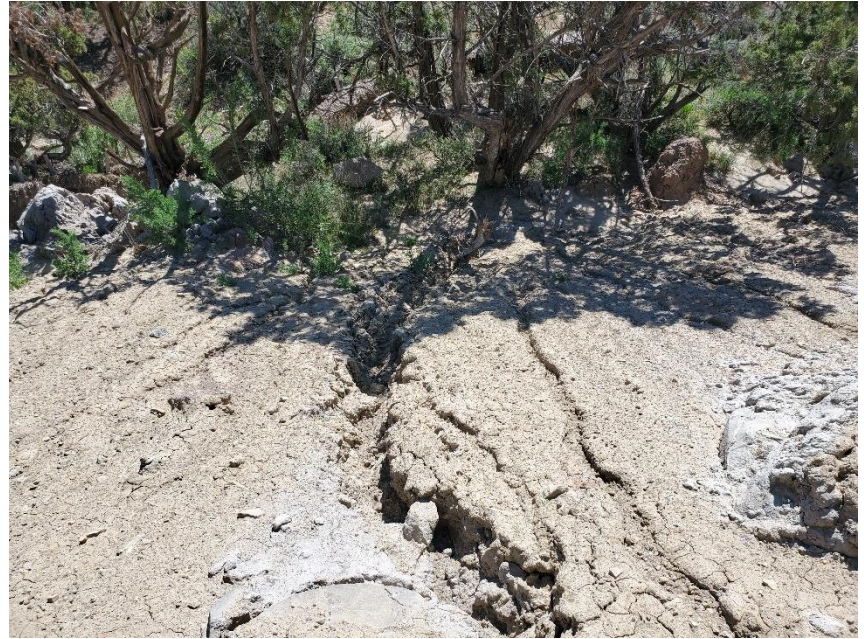
Photo 10: Photo taken from the southeast end of the Location/Location entrance, facing east from the access road. Photo shows erosion degradation and sediment deposition; Insufficient BMPs, or BMPs missing, to stabilize the slopes, manage runoff and prevent degradation to the Location.
