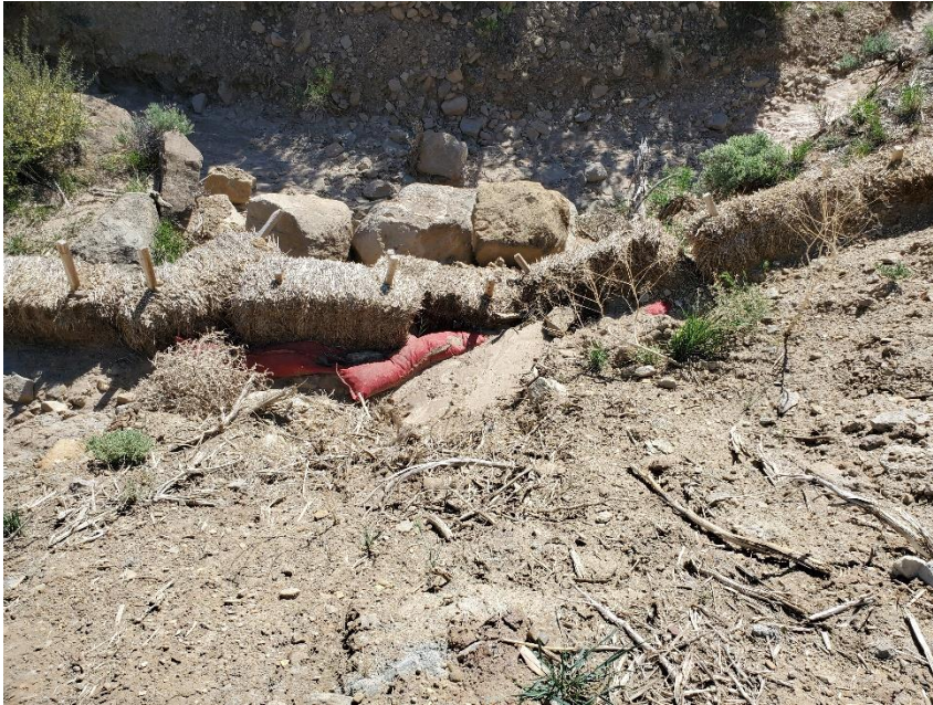
Photo 11: Photo taken from the access road, facing east. Photo shows erosion bales have not been installed in accordance with good engineering practices (entrenched) and/or maintained in proper functioning condition. Sediment discharge into an intermittent stream evident.
