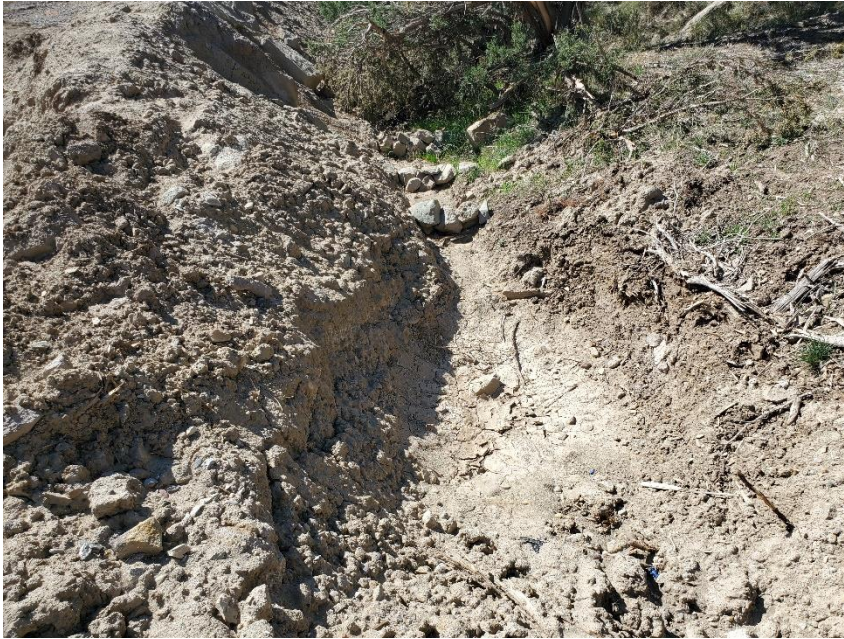
Photo 9: Photo taken from the southwest end of the Location. Photo shows velocity checks within stormwater diversion ditch.
