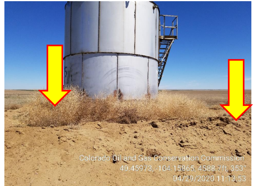
Photo 8 – Tank Berm Integrity, Compromised, Weeds
