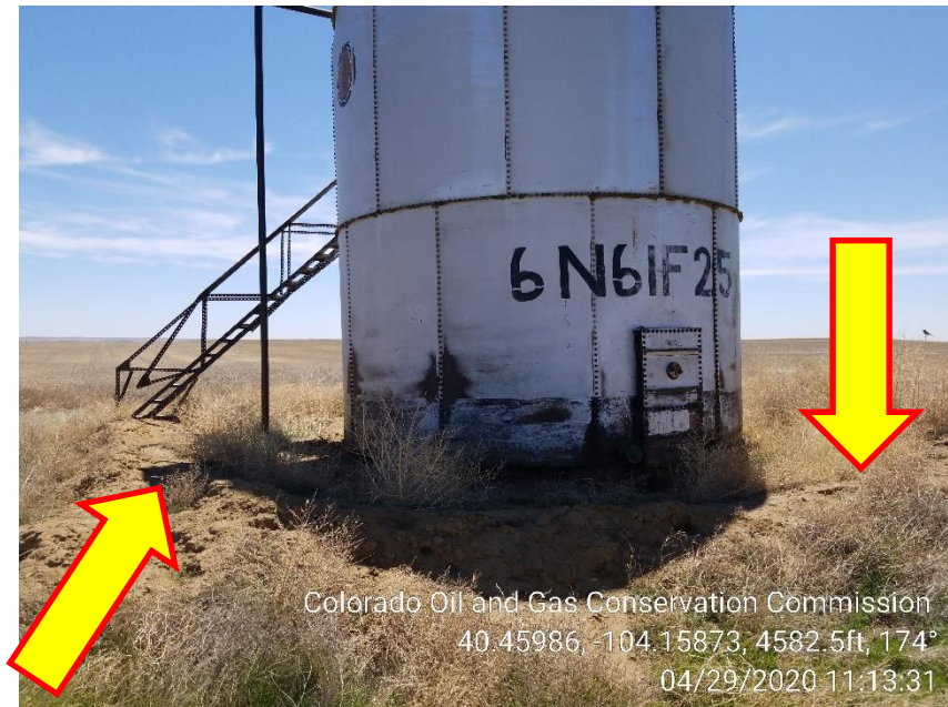
Photo 7 – Tank Berm Integrity, Compromised, Weeds
