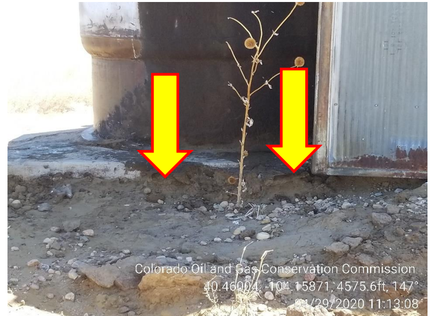
Photo 6 – Stained Soil at Heater Treater
