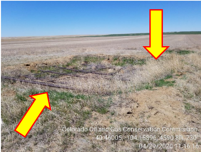
Photo 11 – Pit – Gaps in Mesh, and Weeds
