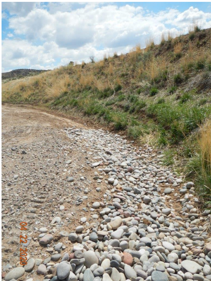
Photo#2: Stormwater repairs.
