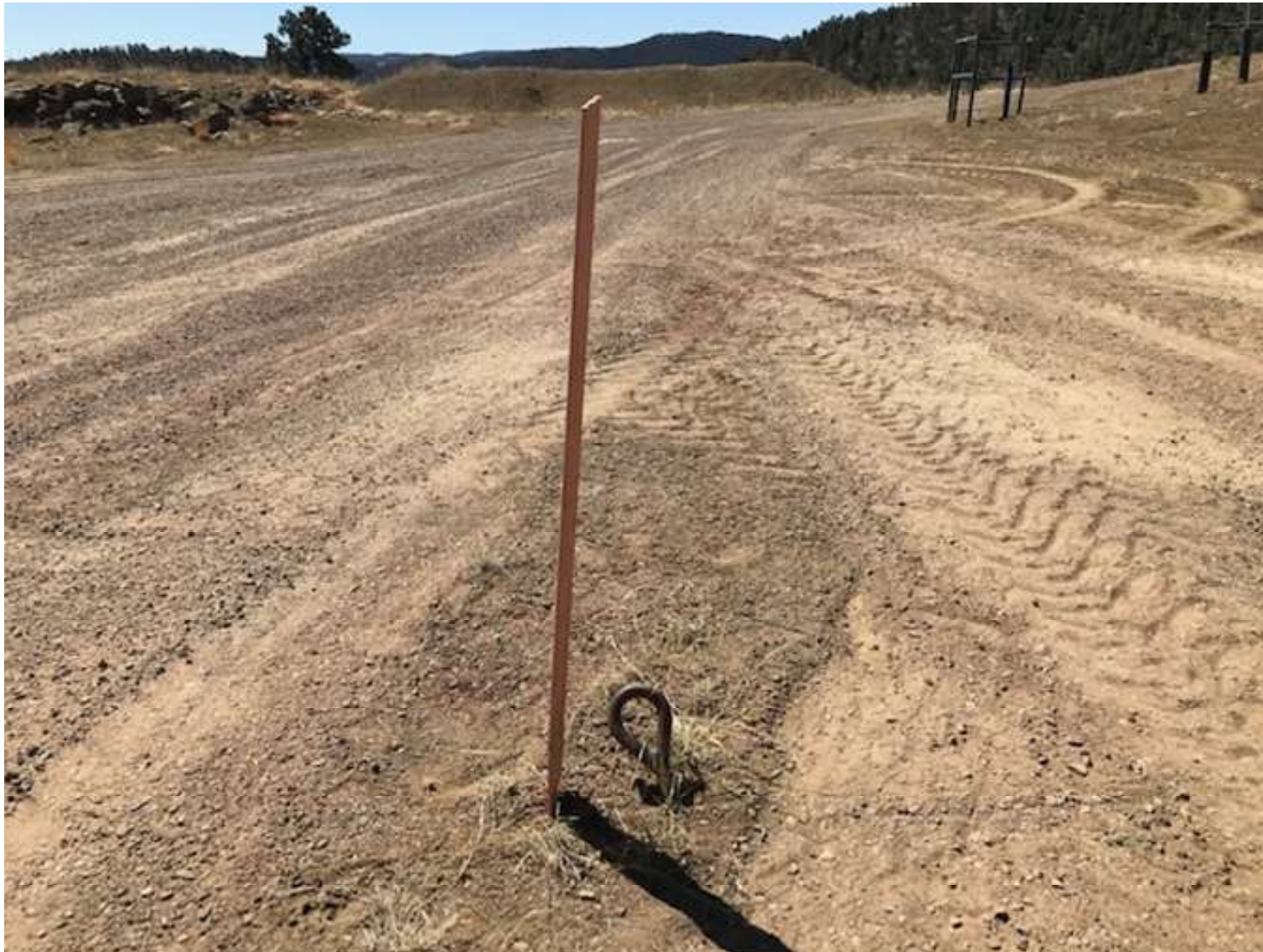
PHOTO 8: THE DOWNED GUY LINE MARKER WAS REINSTALLED.
