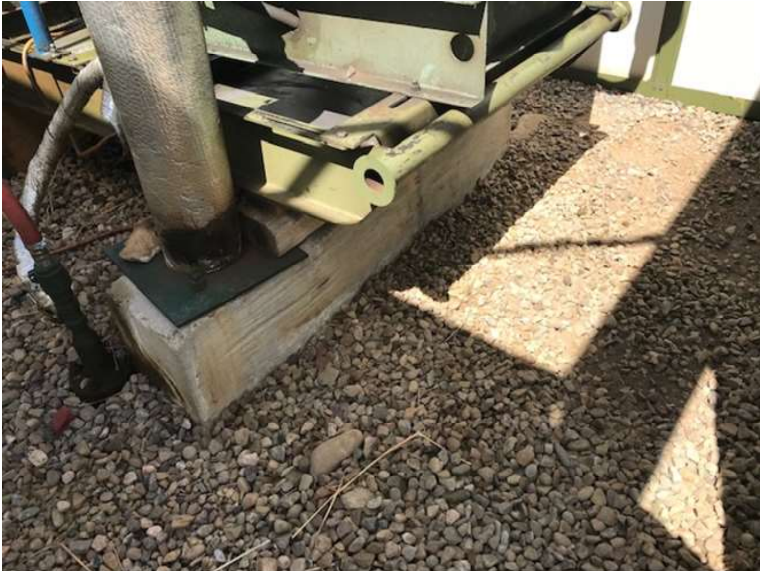
PHOTO 5: THE LEAK ON THE PC ENGINE WAS REPAIRED. THE IMPACTED SOIL/GRAVEL ON THE GROUND WAS CLEANED UP AND REMOVED FROM THE LOCATION.
