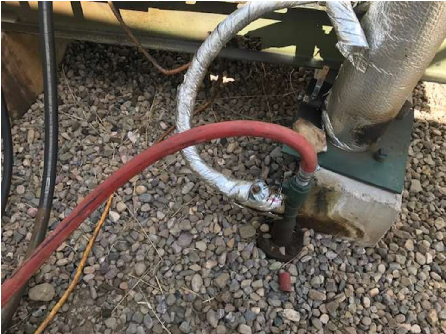
PHOTO 4: THE RED HOSE WAS RE-CONNECTED TO THE WELL HEAD AS THIS IS THE FUEL GAS LINE TO RUN THE PC ENGINE.
