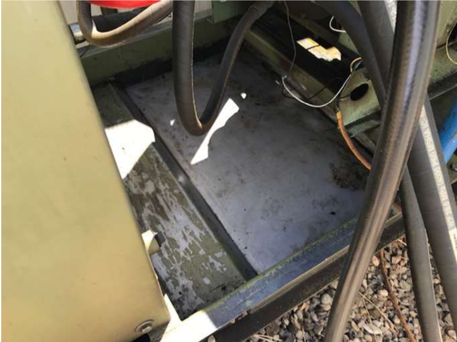
PHOTO 7: THE FLUID ACCUMULATION WAS REMOVED FROM THE CONTAINMENT ON THE PC ENGINE AND THE SKID WAS CLEANED UP.
