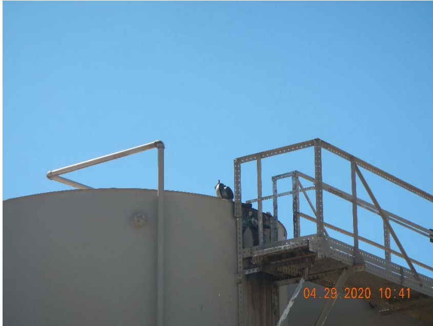
Photo 2. Gauge hatch open on produced water tank.
