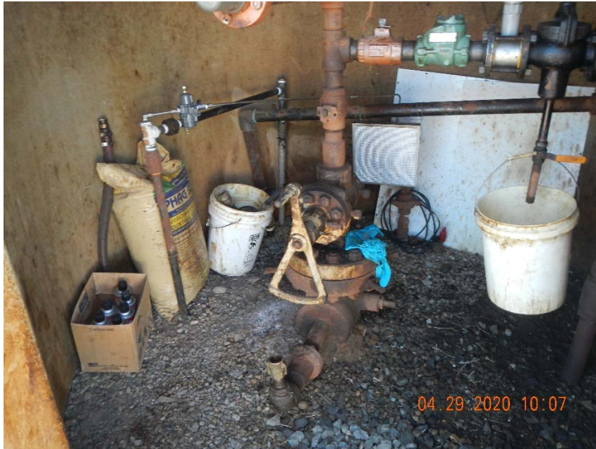
Photo 2. Trash, debris, small equipment stored/discarded inside wellhead housing.
