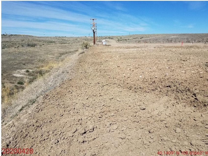
Photo 1: Photo taken from the southeast end of the location, facing west. Photos 1-3 provide an overview of the Location from west, northwest to north. Photos show Operator has constructed a berm between the production area, and areas not needed for production to the east; interim areas have not been contoured to their original grade; fill material has not been removed; Interim reclamation of the Location has not been conducted in accordance with 1003 requirements.
