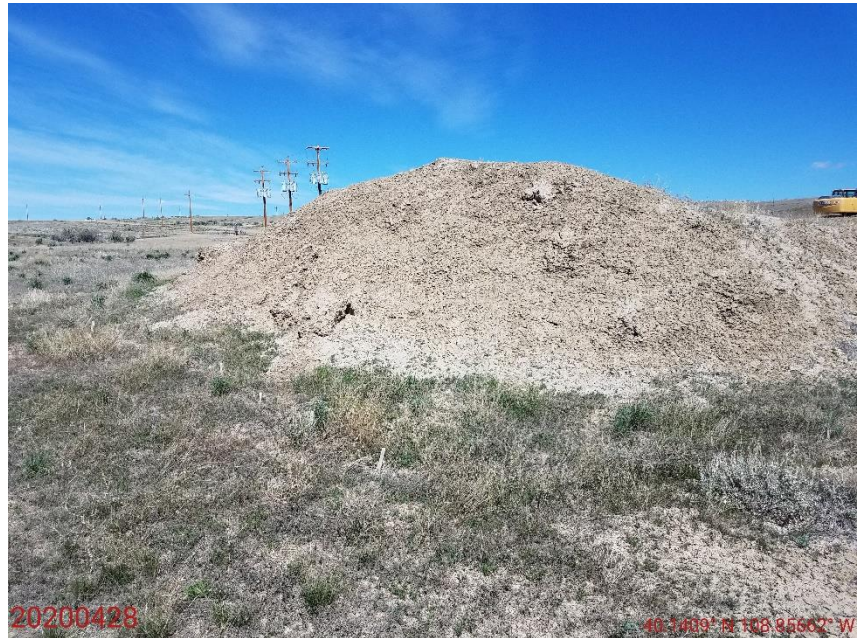
Photo 6: Photo taken from the soil stockpile to the southeast of the Location. Photo shows soils remain bare and exposed; no BMPs have been installed to protect soils in accordance with Rule 1002.c, or to prevent sediment discharge in accordance with Rule 1002.f.
