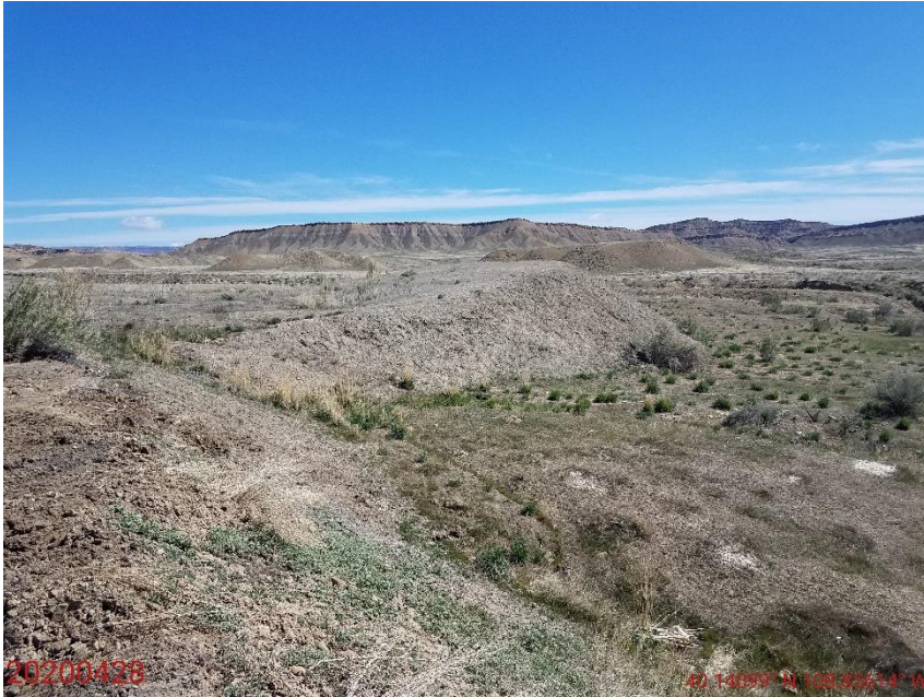
Photo 7: Photo taken from east end of the Location, facing northeast. Photo shows soil stockpile on the northeast end of the Location remains bare and exposed; no BMPs have been installed to protect soils in accordance with Rule 1002.c, or to prevent sediment discharge in accordance with Rule 1002.f.
