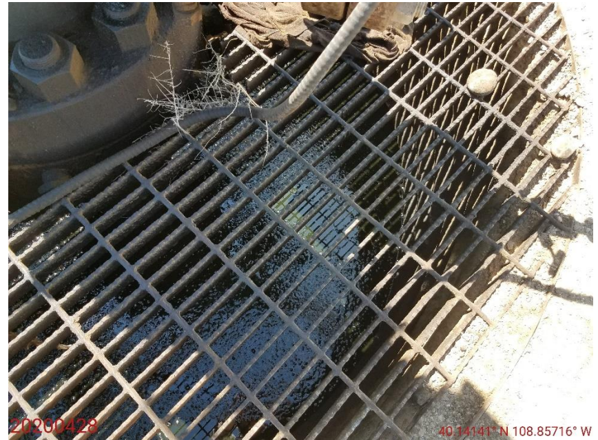
Photo 14: Continued from photo 13. Photo shows oily fluids within the containment cellar; a spill appears to have occurred at well.
