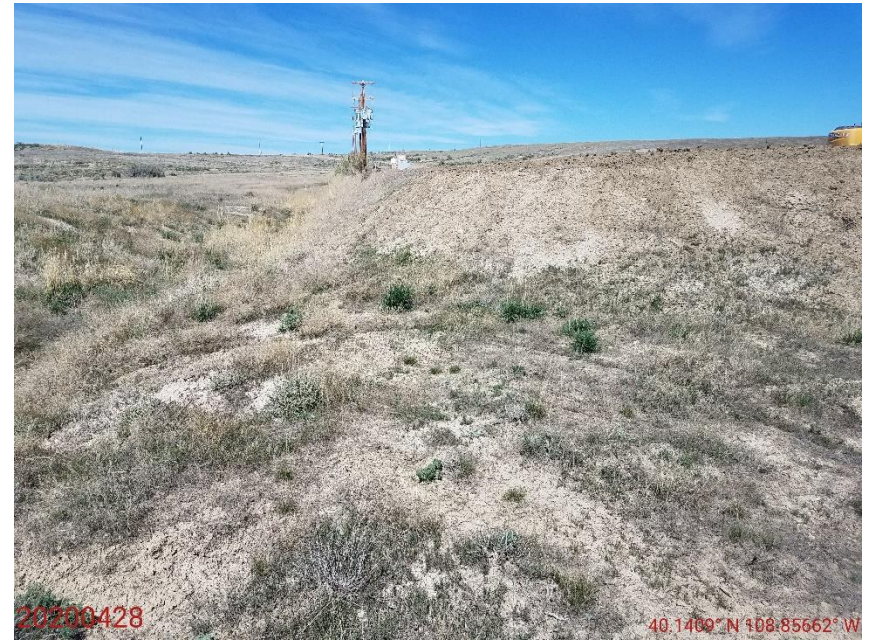
Photo 4: Photo taken from the east of the Location, facing west. Photo shows Operator has not removed fill material on areas subject to 1003 interim reclamation, and lands have not been contoured to their original grade. Interim reclamation of the Location has not been conducted in accordance with 1003 requirements.
