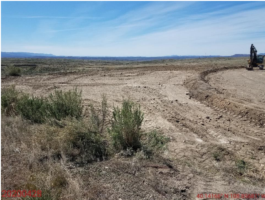
Photo 9: Photo taken from the northeast end of the location, facing south. Photos 1-3 provide an overview of the Location from south, southwest to west. Photos show Operator has constructed a berm between the production area, and areas not needed for production to the east; interim areas have not been contoured to their original grade; fill material has not been removed; Interim reclamation of the Location has not been conducted in accordance with 1003 requirements.
