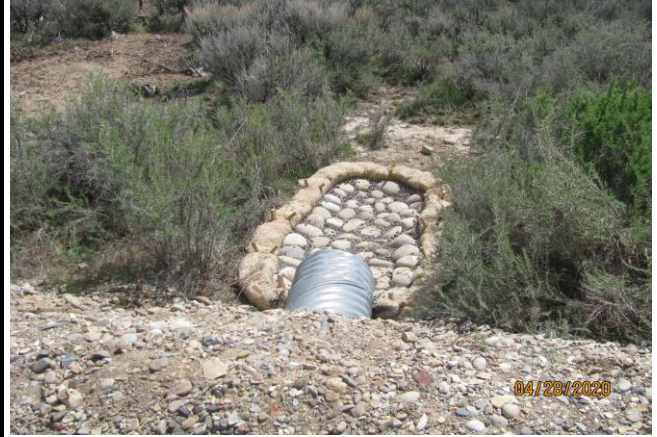
BMPs Installed at Culvert Outlet on the HD 7-23AH Pad
