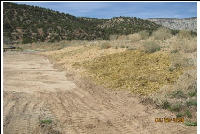
Slope Seeded & Mulched on the NW side of the HD 7-23AH Pad
