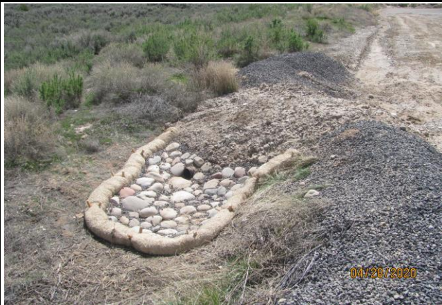
BMPs Installed at Flex Pipe Outlet on the HD 7-23AH Pad
