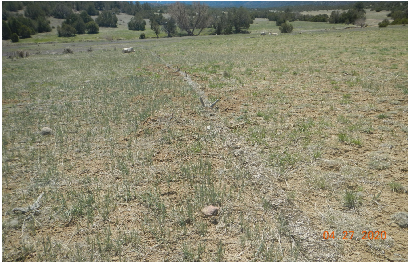
Photo 2. The degraded wattles remain around the eastern perimeter. The degraded wattles and stakes need to be removed.
