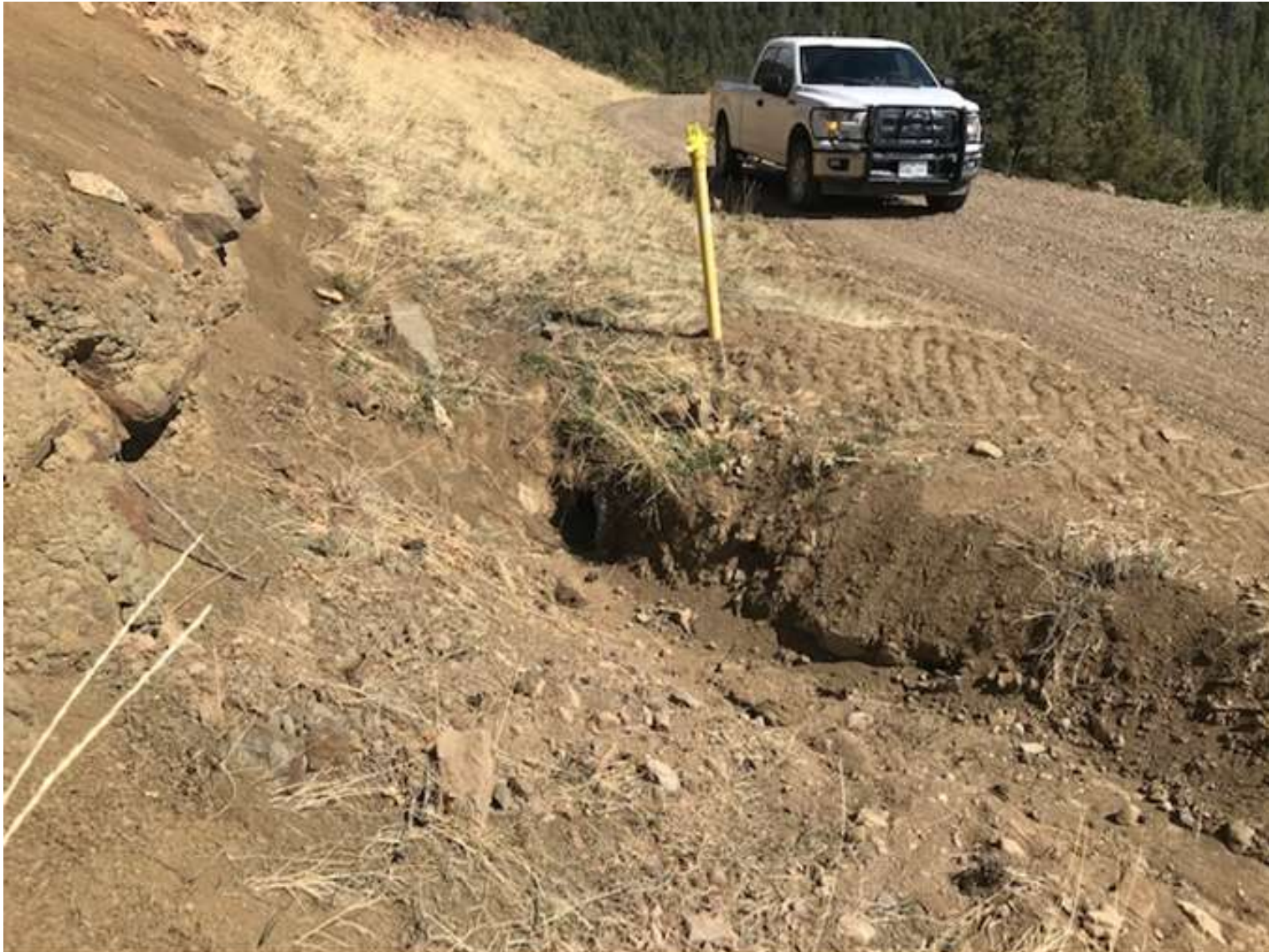
PHOTO 9: THE SEDIMENT ON THE CULVERT INLET ALONG THE MAIN ROAD TOWARD HILL RANCH 1 COMPRESSOR STATION WAS REMOVED.
