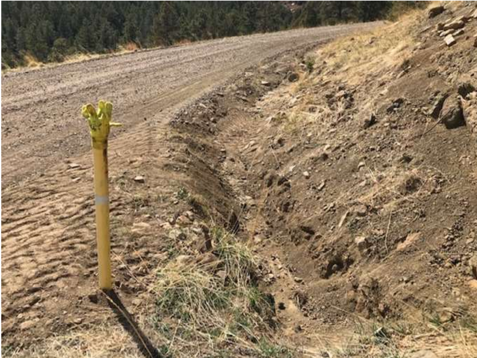
PHOTO 8: THE SEDIMENT ON THE CULVERT INLET ALONG THE MAIN ROAD TOWARD HILL RANCH 1 COMPRESSOR STATION WAS REMOVED.
