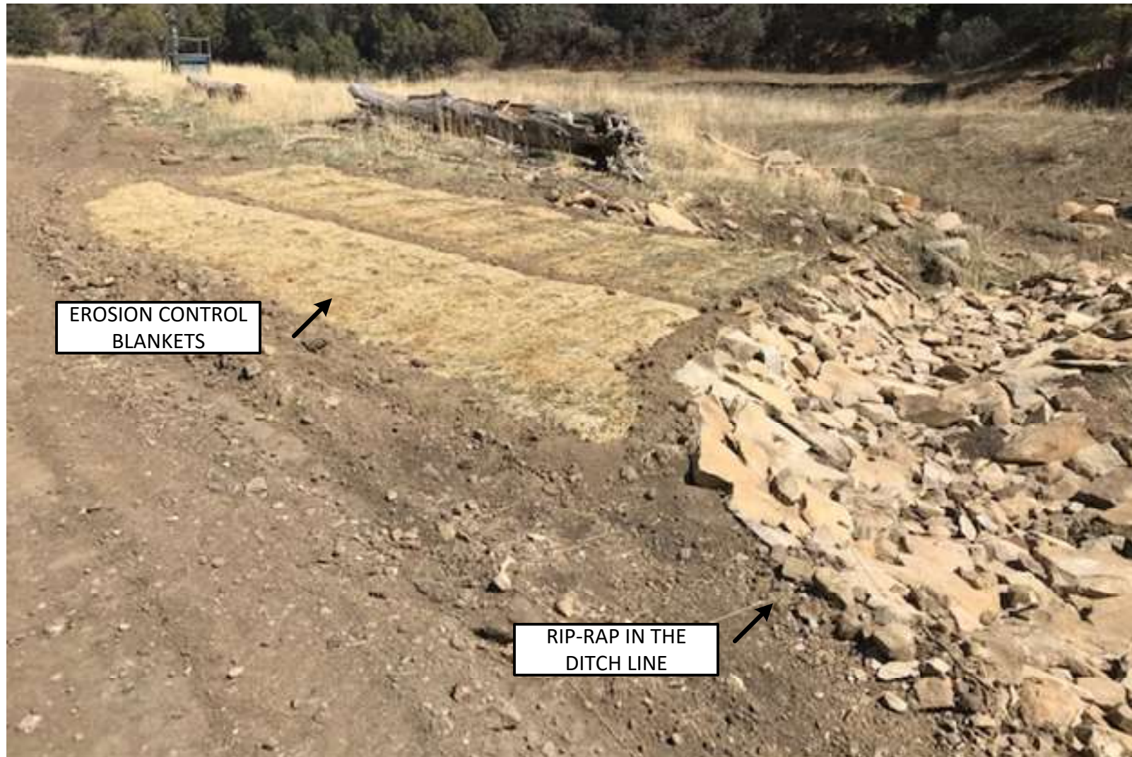
PHOTO 4: THE EROSION ON TOP OF THE CULVERT OUTLET WAS BACK FILLED. THE DISTURBANCE WAS SEEDED WITH AN APPROVED HILL RANCH SEED MIX AND EROSION CONTROL BLANKETS WERE INSTALLED TO STABILIZE THE SOIL. THE EROSION PARALLEL TO THE LEASE ROAD WAS STABILIZED WITH RIP-RAP.
