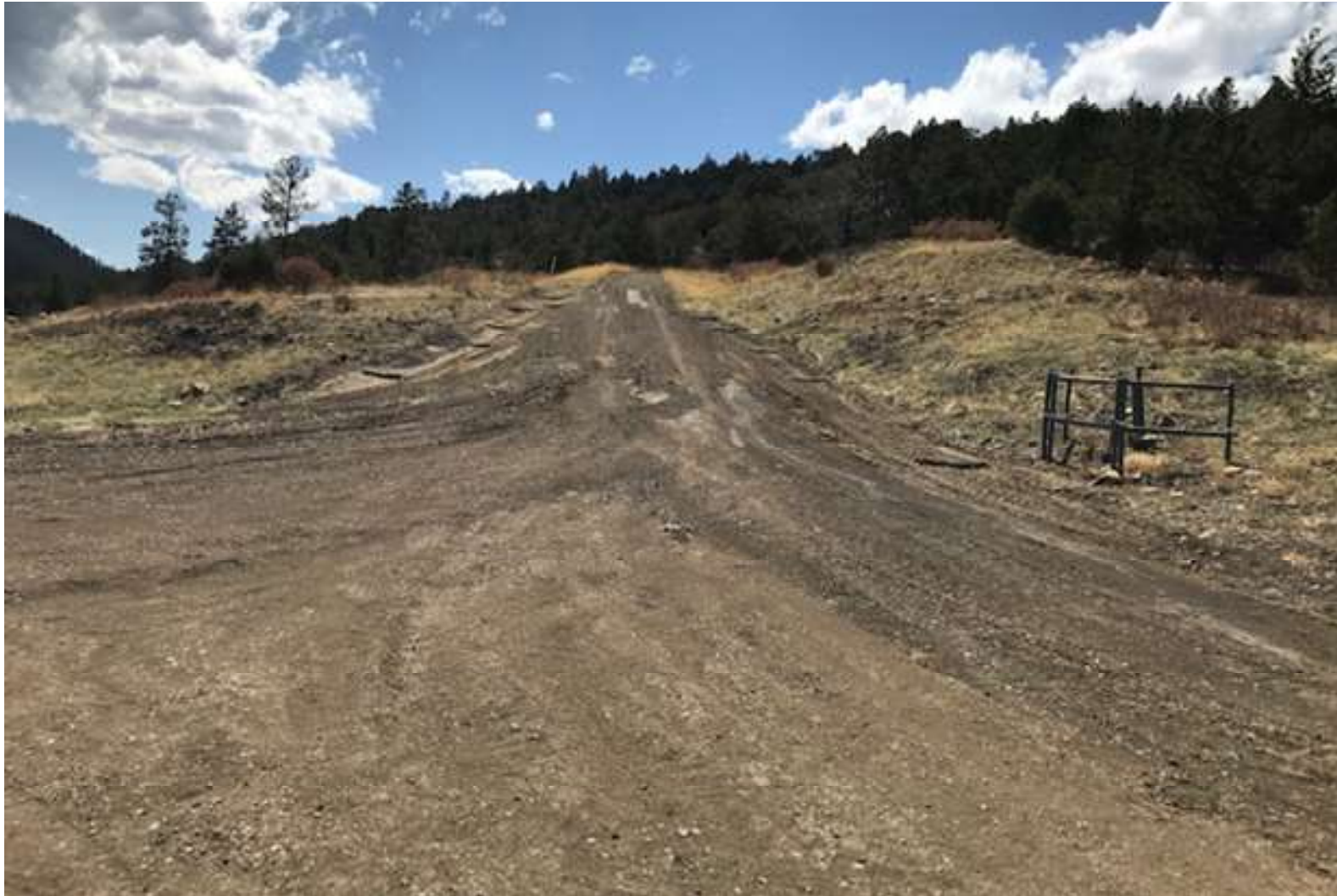
PHOTO 5: THE ACCESS ROAD TO THE LOCATION WAS SURFACE CROWNED TO ESTABLISH SHEET FLOW DURING RUN OFF. THIS ELIMINATED THE TIRE RUTS. THE BAR DITCH ON BOTH SIDES OF THE ACCESS ROAD WERE BACK FILLED AND THE SOIL WAS COMPACTED WITH THE TIRE OF THE BACKHOE FOR SOIL STABILIZATION AND TO ELIMINATED THE DITCH CUTTING.
