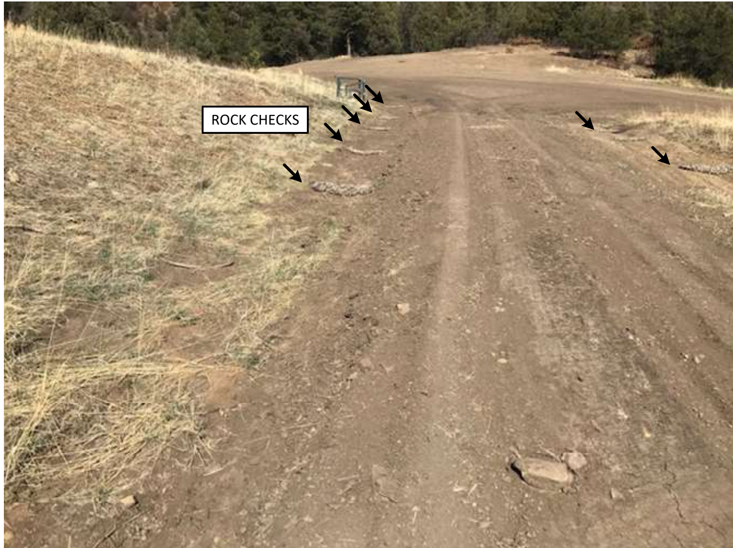
PHOTO 6: ROCK- SOCK CHECK DAMS WERE PLACED IN THE BAR DITCH ON BOTH SIDES OF THE ACCESS ROAD.
