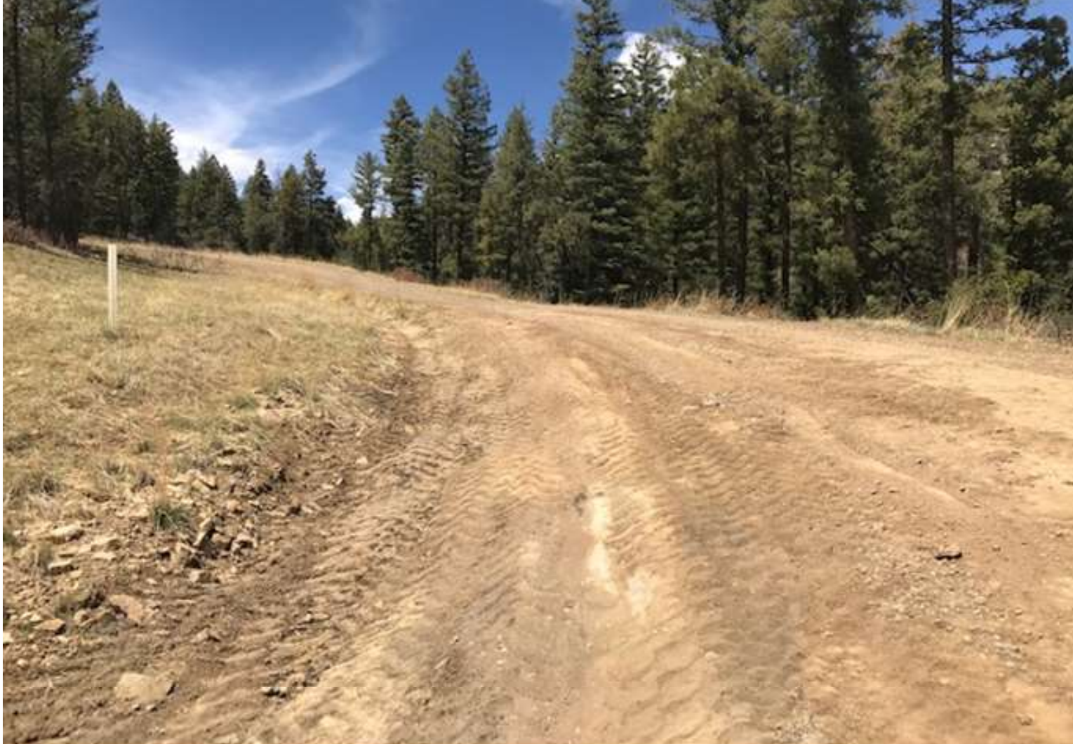
PHOTO 7: THE BAR DITCH WAS BACK FILLED AND THE SOIL WAS COMPACTED WITH BACK HOE TIRE TO ELIMINATED THE DITCH CUTTING ALONG THE MAIN ROAD.
