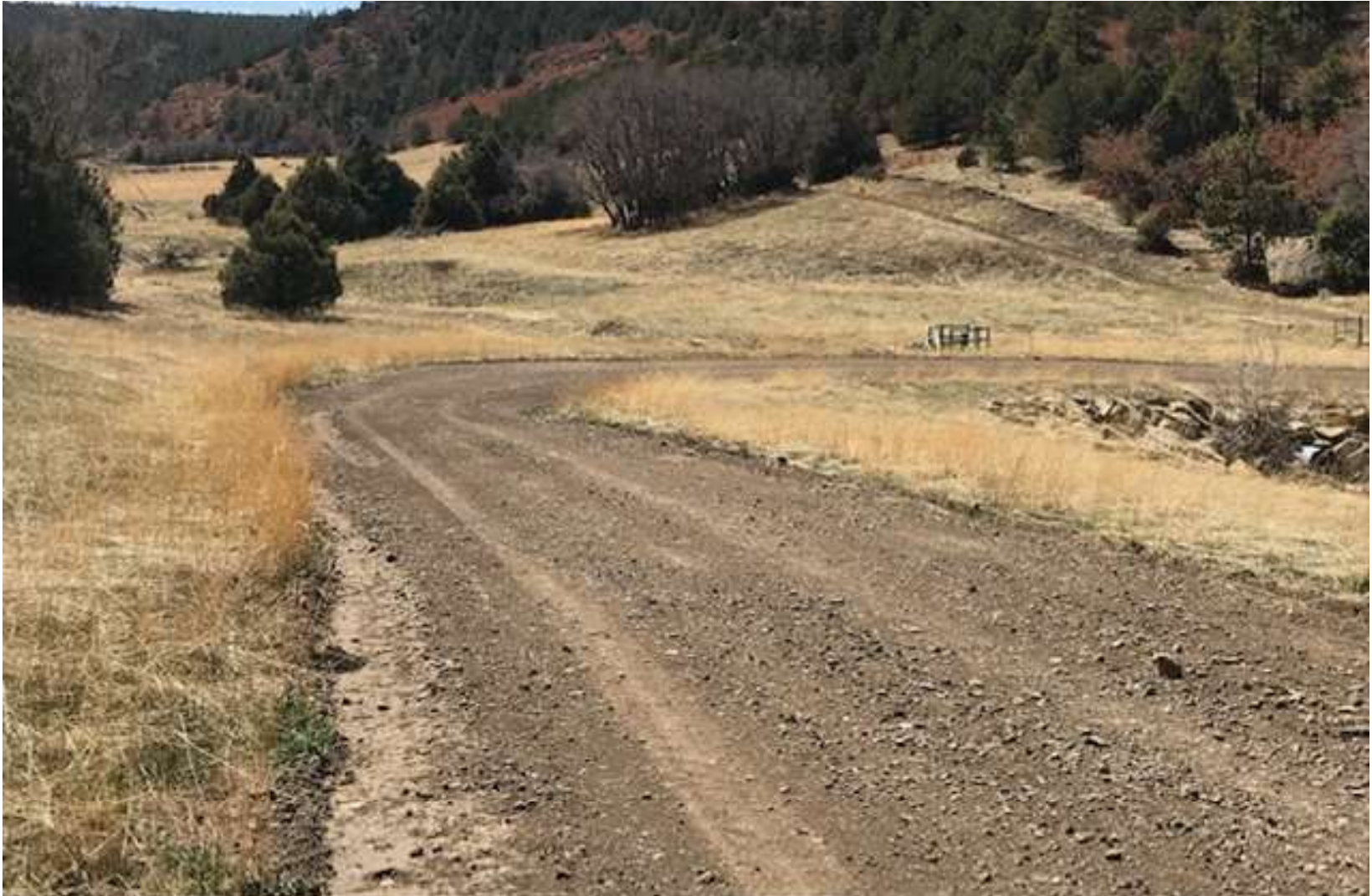
PHOTO 3: THE LEASE ROAD WAS SURFACE CROWNED TO ESTABLISH SHEET FLOW DURING RUN OFF. THIS ELIMINATED THE CONCENTRATED FLOW FOUND IN THE TIRE RUTS.
