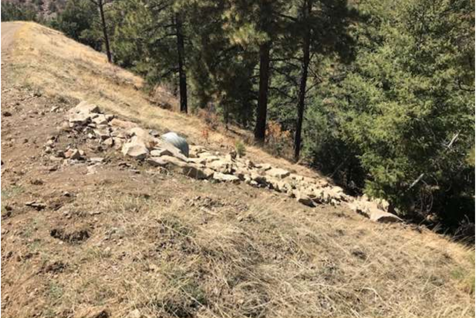
PHOTO 2: THE EROSION ON THE SAME CULVERT OUTLET ON THE MAIN ROAD WAS REPAIRED AND STABILIZED WITH RIP RAP FOR EROSION CONTROL.
