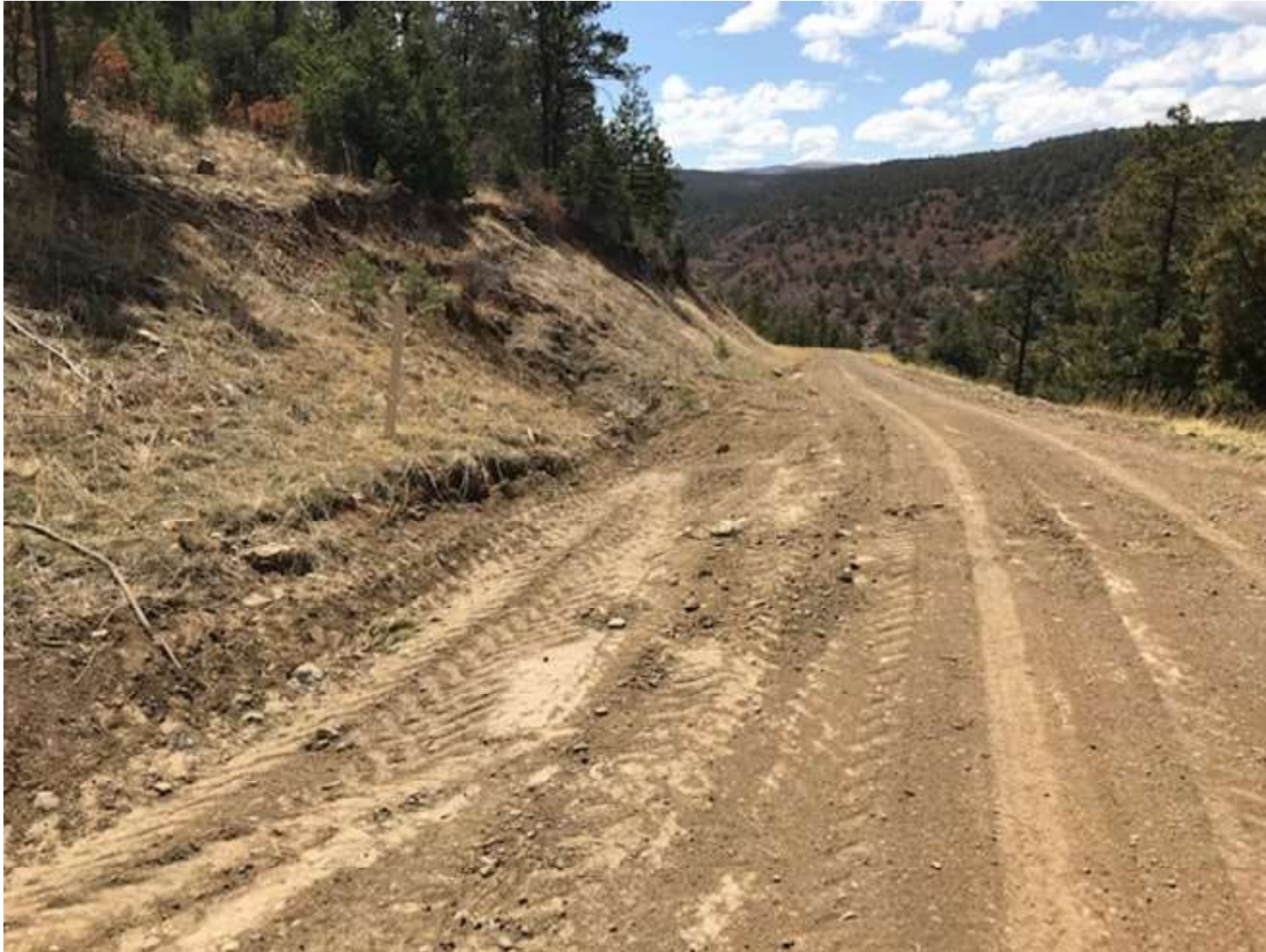
PHOTO 1: THE BAR DITCH WAS BACK FILLED AND THE SOIL WAS COMPACTED WITH THE TIRE OF THE BACKHOE FOR SOIL STABILIZATION AND TO ELIMINATED THE DITCH CUTTING ALONG THE MAIN ROAD. THE SNOW COVER HAS MELTED AND THE CULVERT INLET DOES HAVE FLOW.
