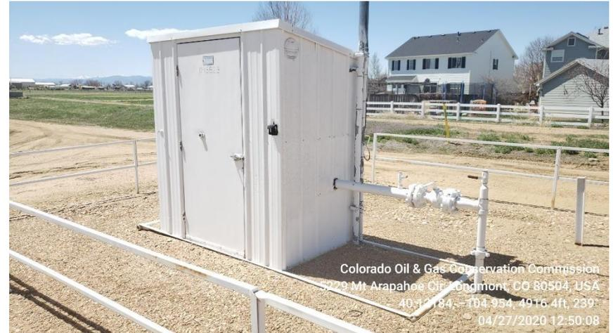
**Photo 7 Horizontal Heated Separator**
