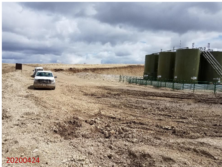
Photo 21: Photo taken from the west end of the Location, facing northeast. Photo shows stormwater ponding on the Location; Pad does not appear to have been constructed in such a manner to allow for proper stormwater discharge from the location; this does not comport with 1002.f
