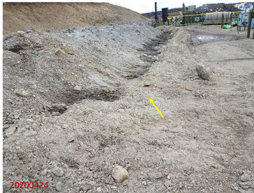
Photo 20: Photo taken from the northwest corner of the Location, facing east. Photo shows area of the berm along the drill cuttings in disrepair.
