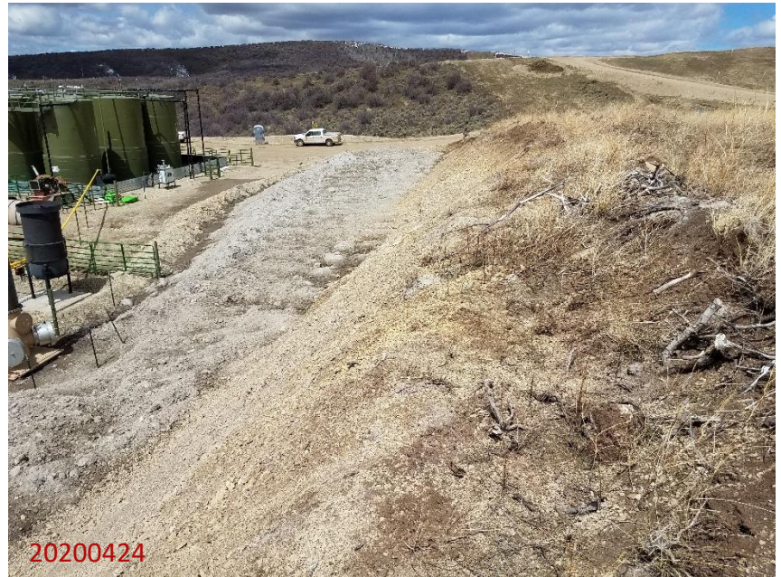
Photo 18: Photo taken from the cut slope on the north end of the Location. Photo shows cut slopes are predominantly exposed; stabilization BMPs missing.
