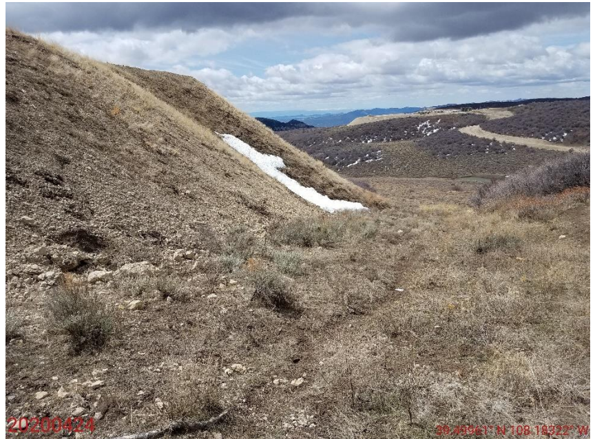
Photo 6: Photo taken from the northwest perimeter of the disturbance area, facing south. Photo shows fill slopes are predominantly exposed, or vegetated by undesirable weedy annual species (cheat grass). Photo also shows perimeter stormwater BMPs missing.
