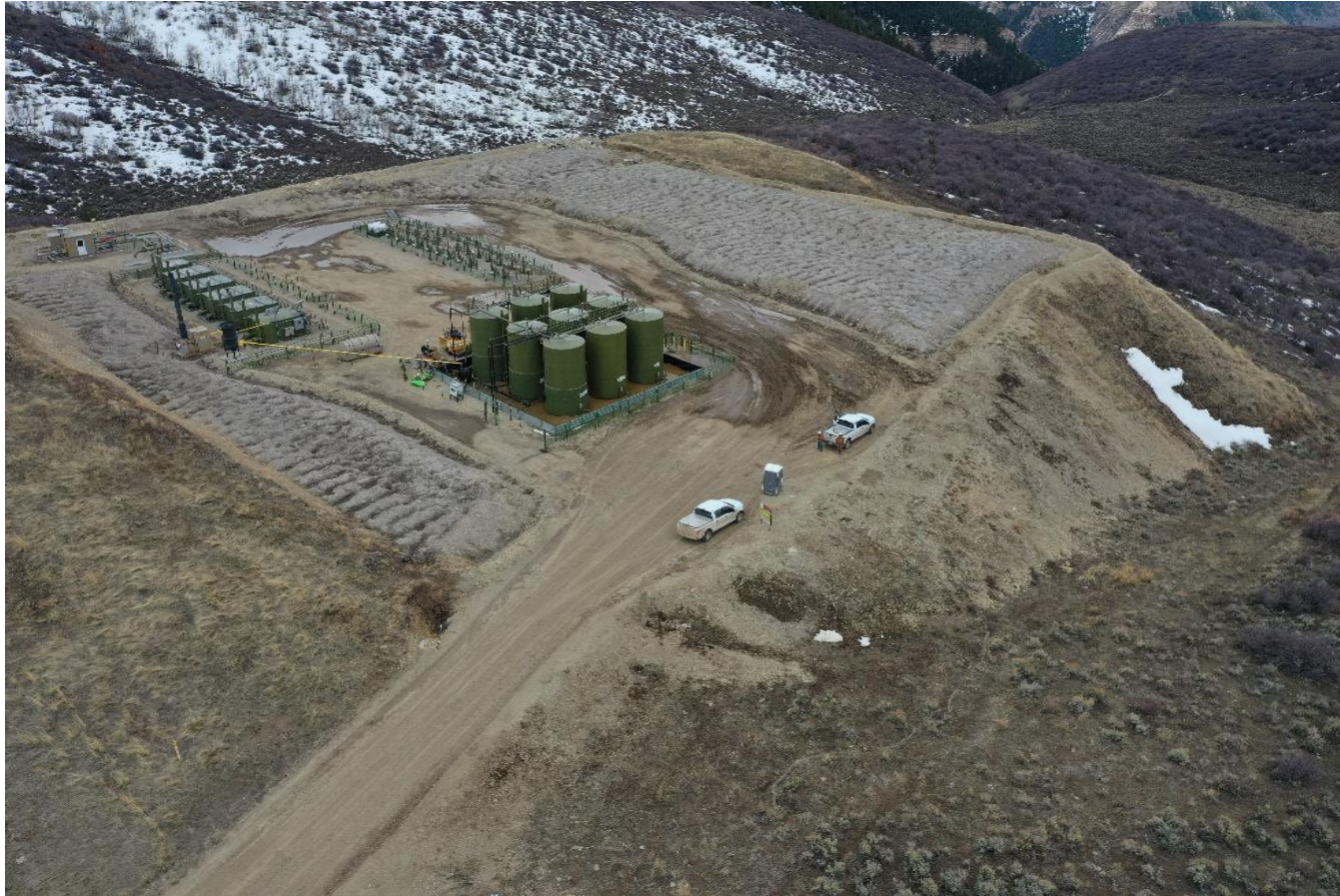
Photo 30: On 4/24/2020, Reclamation specialist Trujillo utilized a SUA to capture an aerial image of the Location; Photo taken from the northwest end of the Location, facing southeast. See comments under photo 29. Photo also show fill slopes on the west end of the location are predominantly exposed. Photo also shows perimeter BMPs are either in disrepair, or missing.
