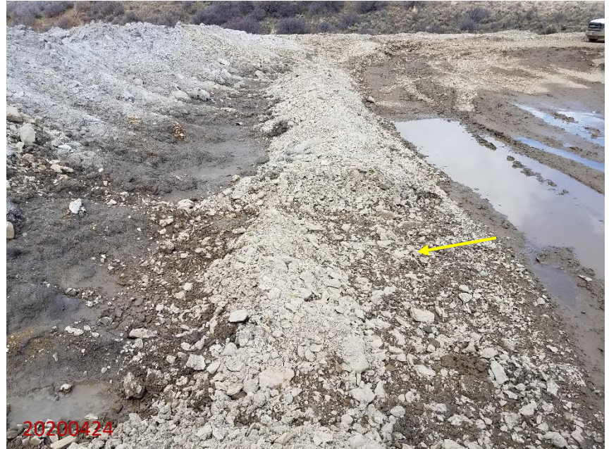
Photo 28: Photo taken from the south end of the Location, facing west. Photo shows area of the berm along the drill cuttings in disrepair.
