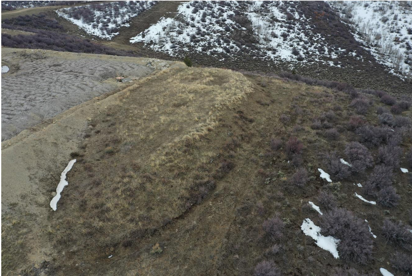
Photo 34: Photo of topsoil pile on the south end of the Location. Photo also show fill slopes on the west end of the location are predominantly exposed. Photo also shows perimeter BMPs are either in disrepair, or missing.
