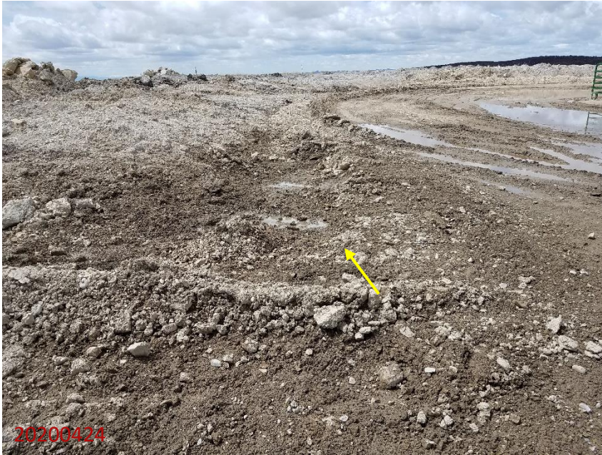
Photo 27: Photo taken from the northeast corner of the Location, facing south. Photo shows area of the berm along the drill cuttings in disrepair.
