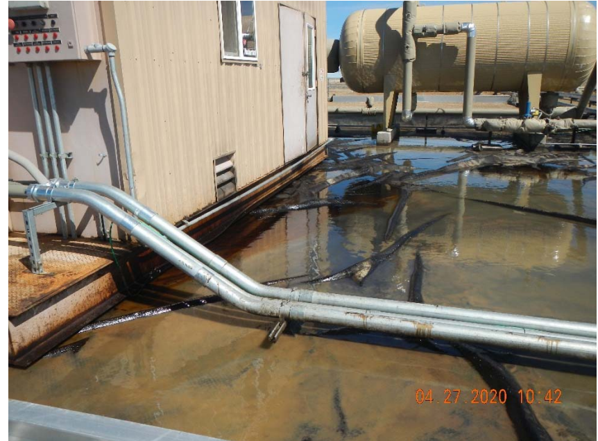
Photo 2. E&P waste fluid in jet pump secondary containment.
