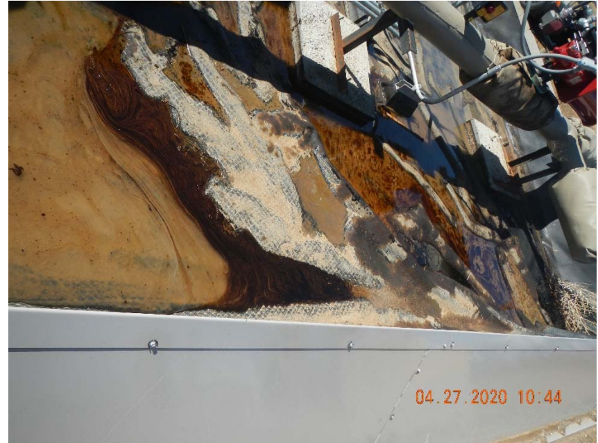
Photo 4. E&P waste fluid in jet pump secondary containment.
