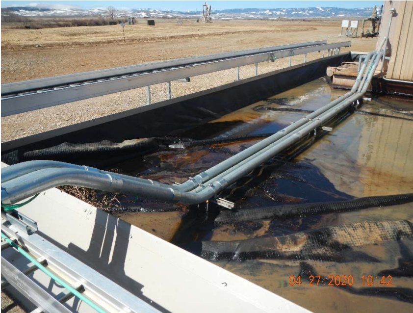
Photo 3. E&P waste fluid in jet pump secondary containment.
