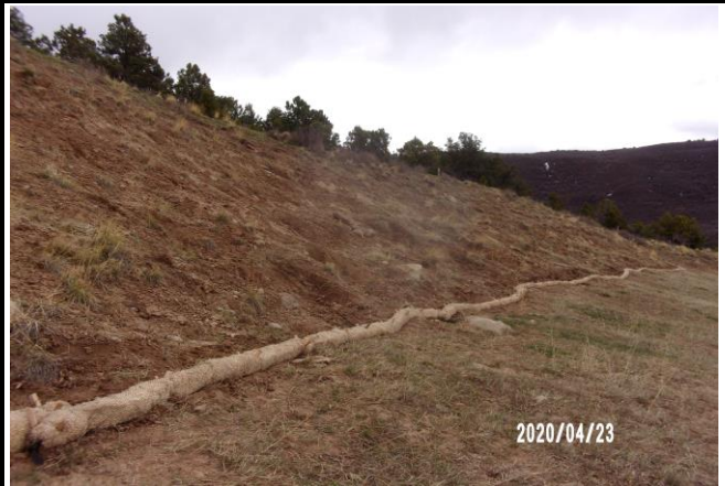
Wattle Installed at the Base of the Cut Slope on the Hidden Creek 14-14 Pad
