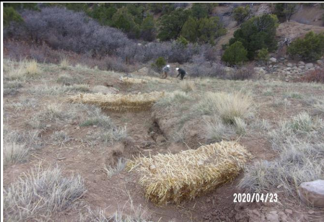
Additional BMPs Installed within Dewatering Channel on the Hidden Creek 14-14 Pad
