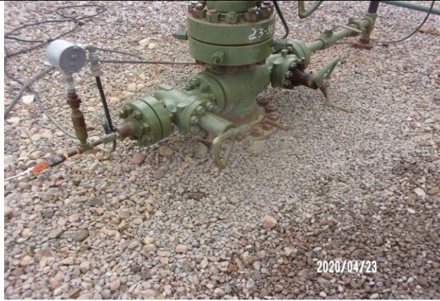
Stained Soil Cleaned Up at the Well Head on the Hidden Creek 14-14 Pad
