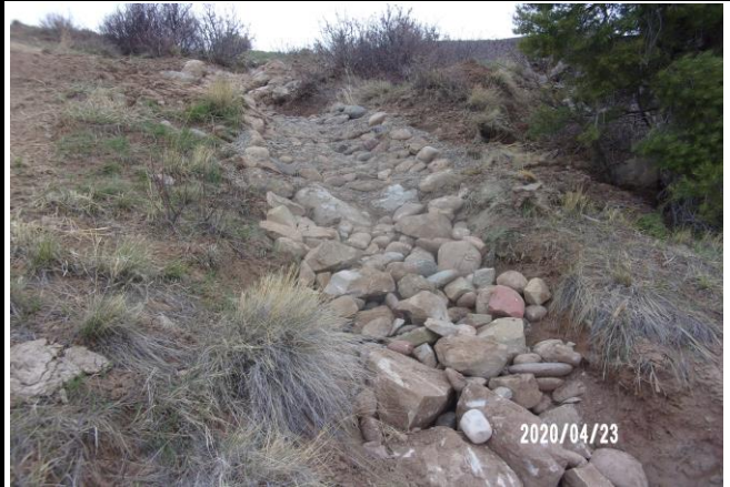
Rock Apron Outlet Repaired on the Fill Slope of the Hidden Creek 14-14 Pad
