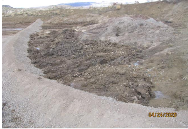
Containment Berm Installed around the Cuttings Pile in the SE Corner of the Hells Gulch 26-11 Pad
