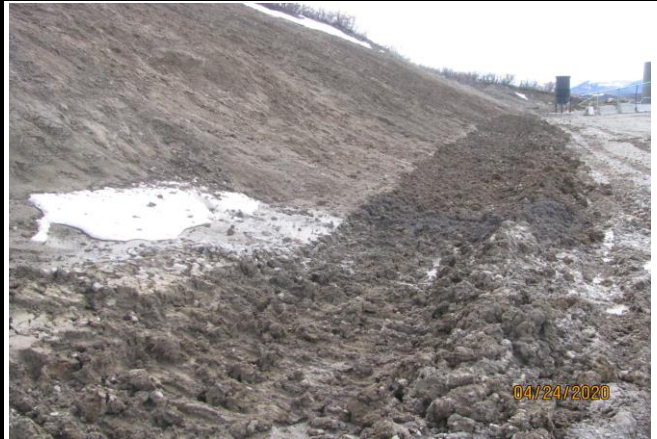
Berm Installation along the Cut Slope on the Hells Gulch 26-11 Pad
