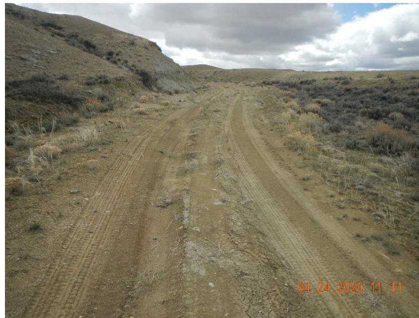
Photo 4. Apparent sediment migration down access road.
