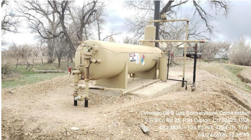
**Photo 9 Horizontal Heated Separator**
