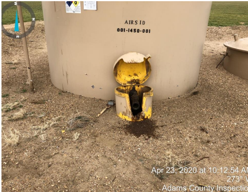
Photo#3 Bullplug missing/Stained soil around load line bucket
