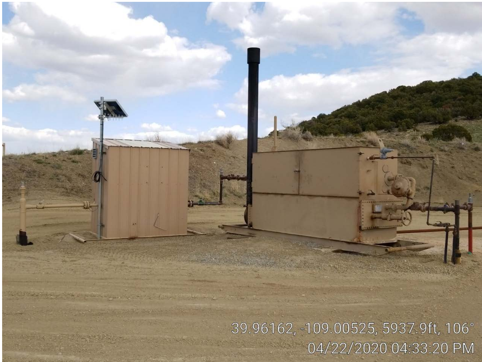
Photo 3. Meter building & separator.
