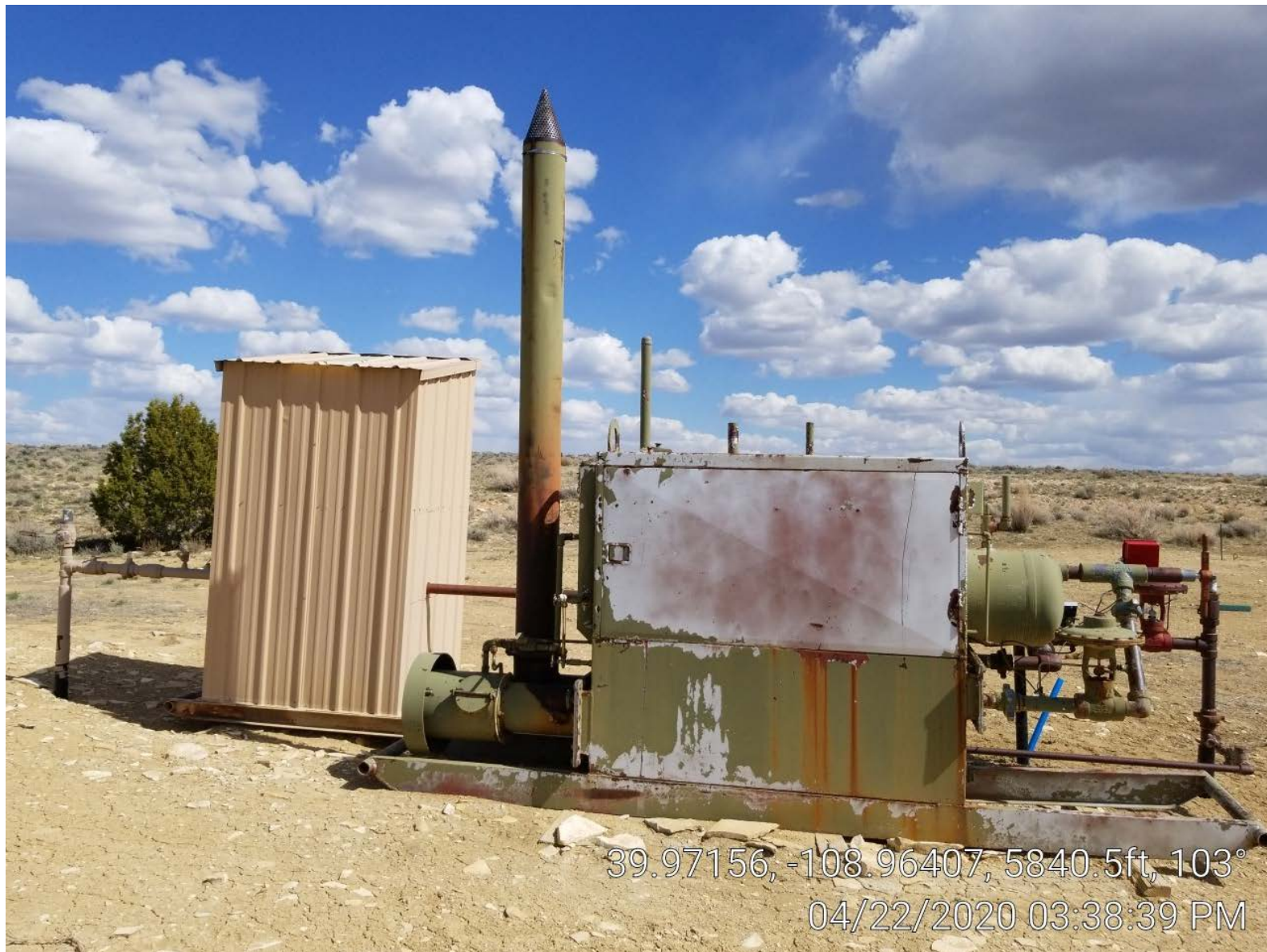
Photo 2. Meter building & separator.
