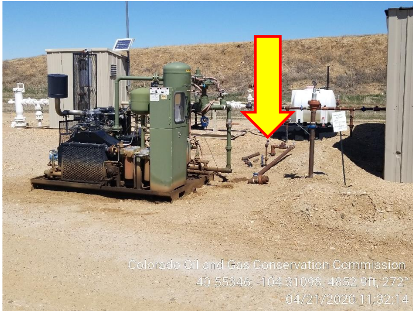
Photo 3 – Unmarked Risers at VRU
