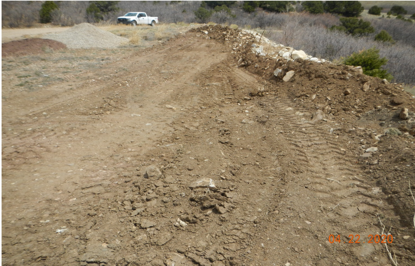
Photo 6. There is pile of soil material being stored and removed at the east side of the location. This should be leveled and reseeding. This issue is disturbing the location.
