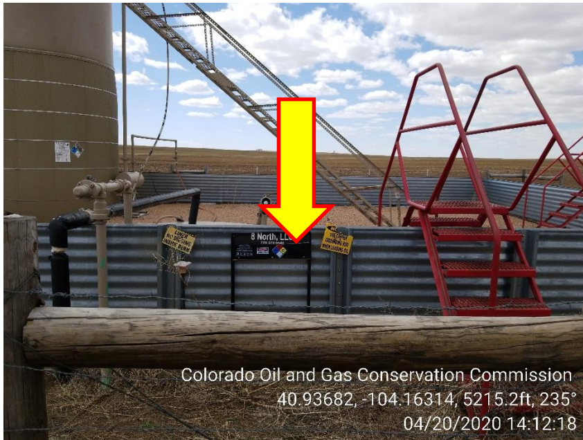
Photo 3 – Produced Water Vault missing Capacity Label
