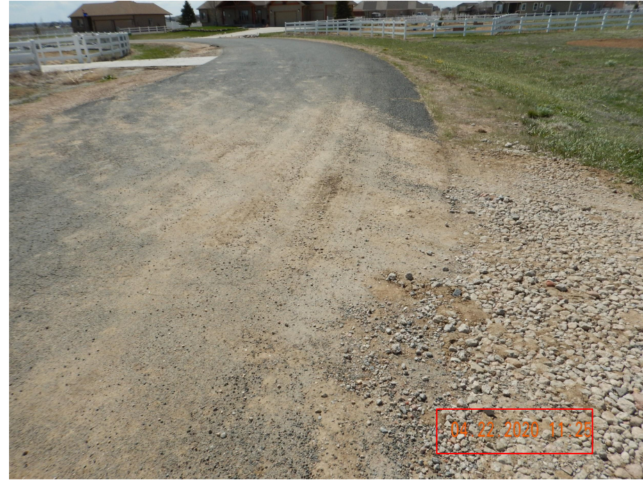
Photo 3. Photo taken from the entrance of location on April 22, 2020, facing South along Lansing Ct. Photo illustrates Operator did minimal to no clean up from vehicle tracking on Lansing Ct.
