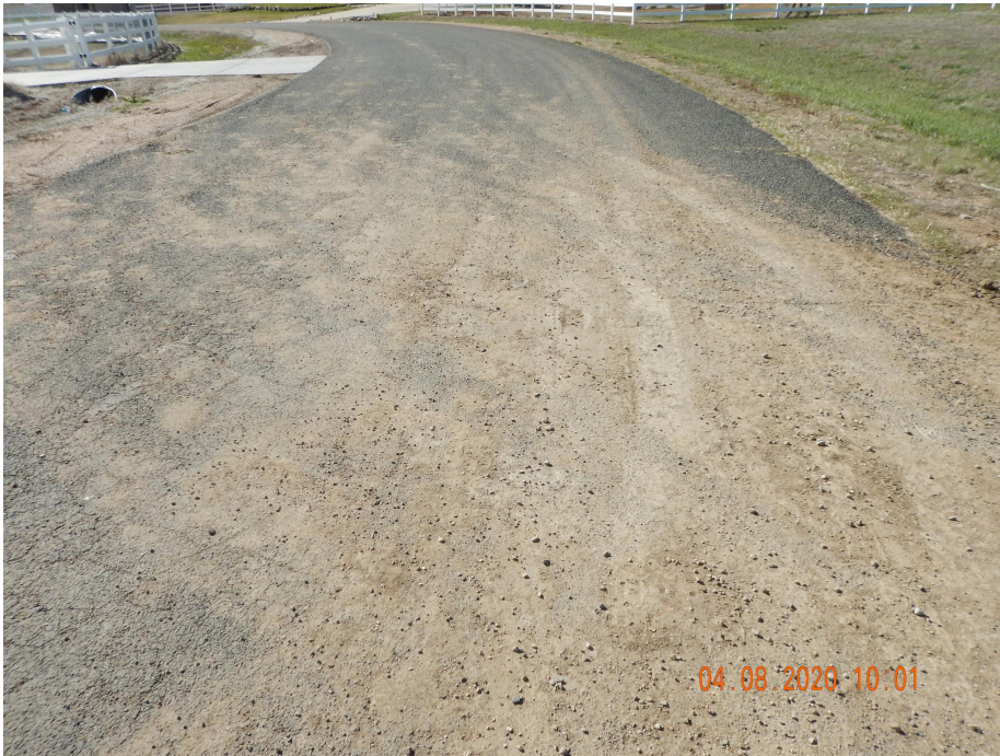
Photo 2. Photo taken from the entrance of location on April 8, 2020, facing South along Lansing Ct. Photo illustrates sediment discharge from vehicle tracking on Lansing Ct.
