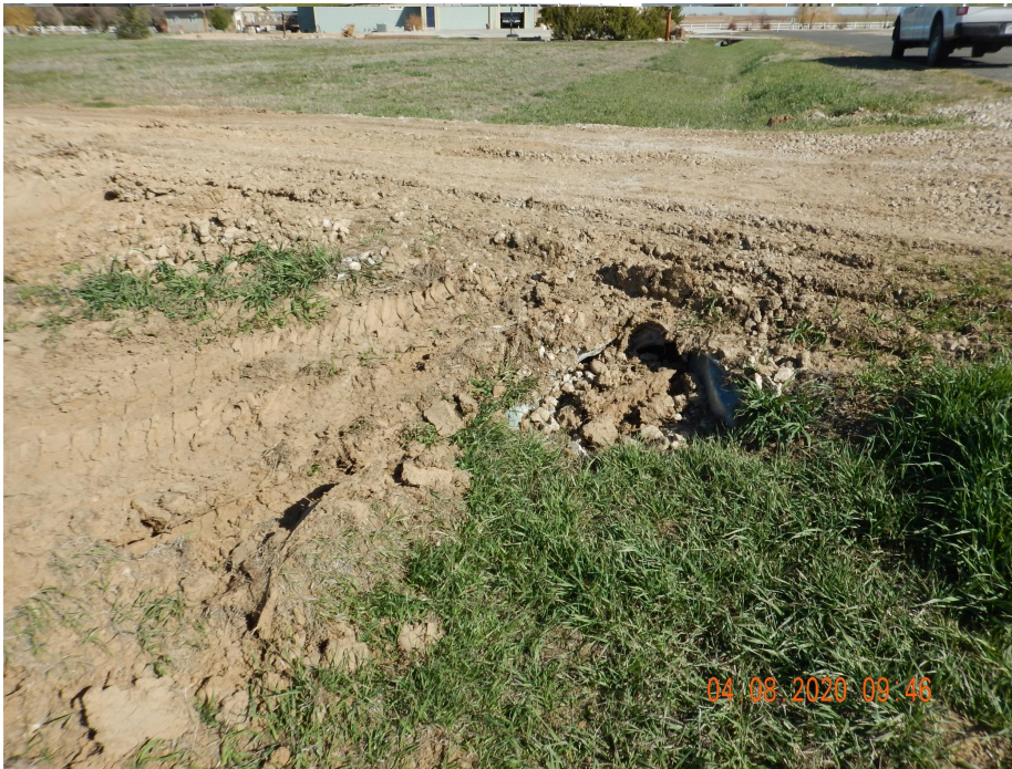
Photo 4. Photo taken from the entrance of location on April 8, 2020, facing North. Photo illustrates a damaged culvert from vehicle traffic.
