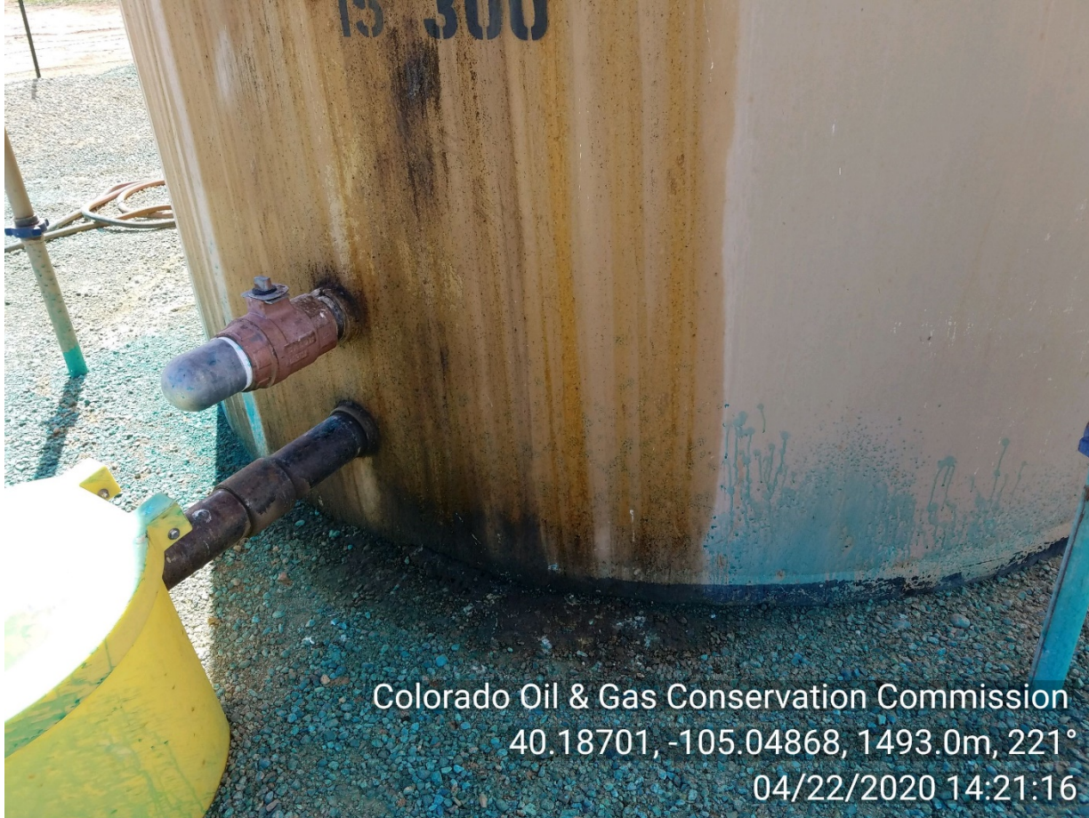
Fluid on front of tank and soil
