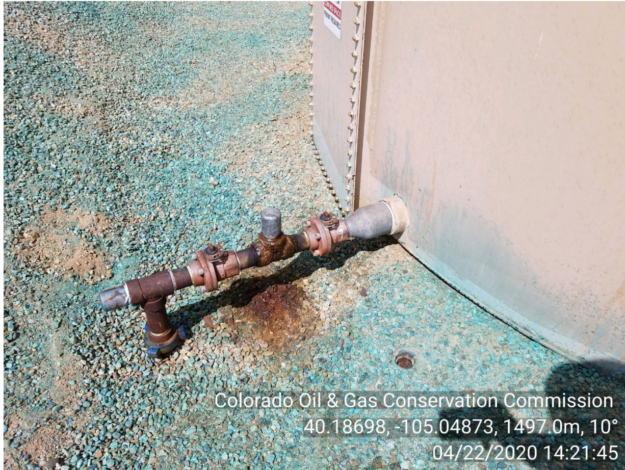
Fluid on backside drain valve and soil
