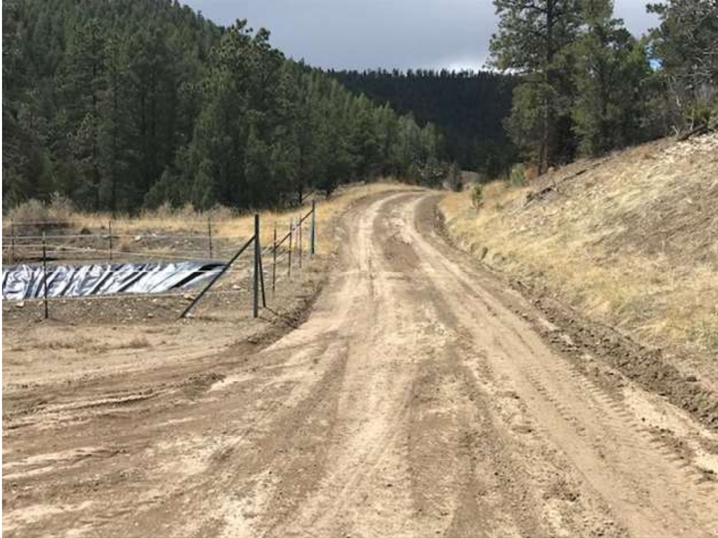
PHOTO 1: THE MAIN LEASE ROAD WAS SURFACE CROWNED TO ESTABLISH SHEET FLOW AND ELIMINATE THE TIRE RUTS.
