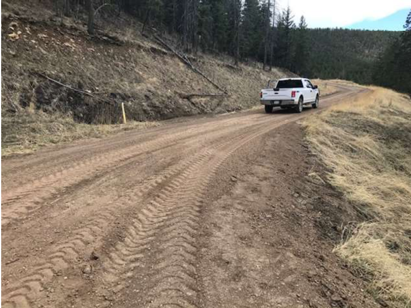
PHOTO 3: THE SEDIMENT ACCUMULATION WAS REMOVED FROM THE CULVERT INLET ALONG THE MAIN LEASE ROAD. SHEET FLOW WAS ESTABLISHED ALONG THE LEASE ROAD TO ADDRESS THE EROSION ISSUES.
