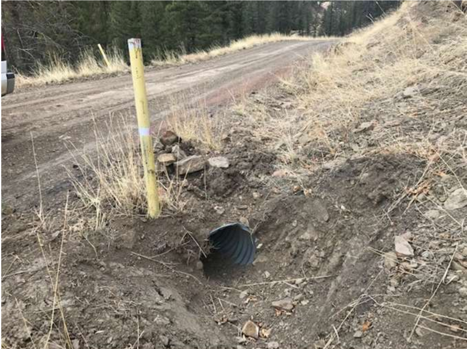
PHOTO 4: THE SEDIMENT ACCUMULATION WAS REMOVED FROM THE CULVERT INLET ALONG THE MAIN LEASE ROAD.
