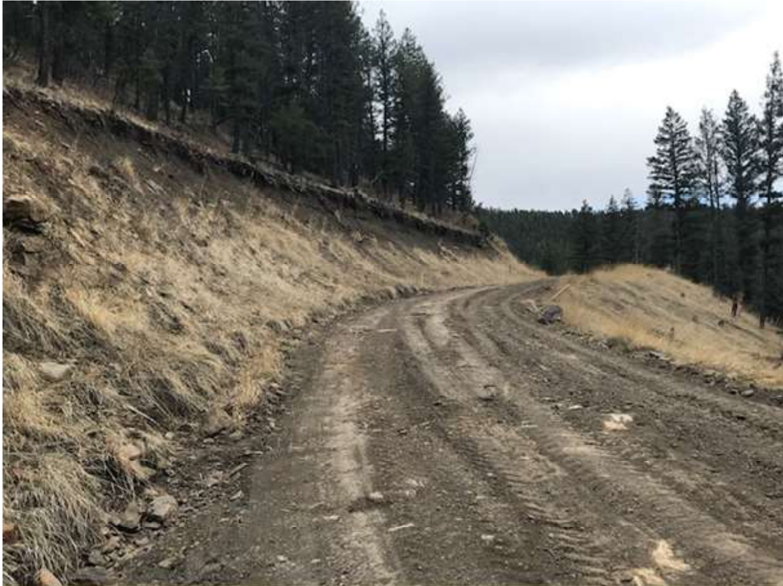
PHOTO 2: THE MAIN LEASE ROAD WAS SURFACE CROWNED TO ESTABLISH SHEET FLOW AND ELIMINATE THE TIRE RUTS. THE LARGE ROCK WAS REMOVED FROM THE DRIVING SURFACE.
