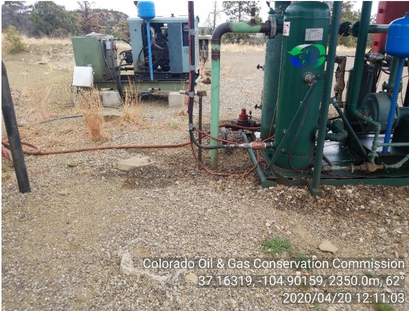
PHOTO 7: AREA OF IMPACTED SOIL AROUND COMPRESSOR SKID. Conduct maintenance on equipment, cleanup stained material and review self inspection processes. CA DATE 4-25-20.
