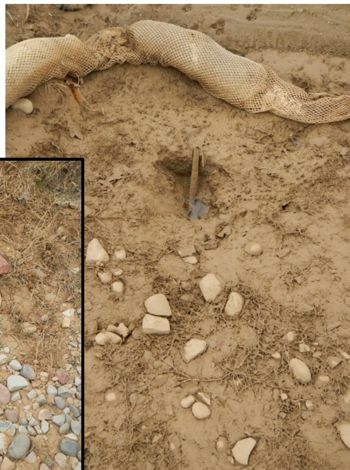
Photo#11: Blocked drains on Pad Fill slope edge.
