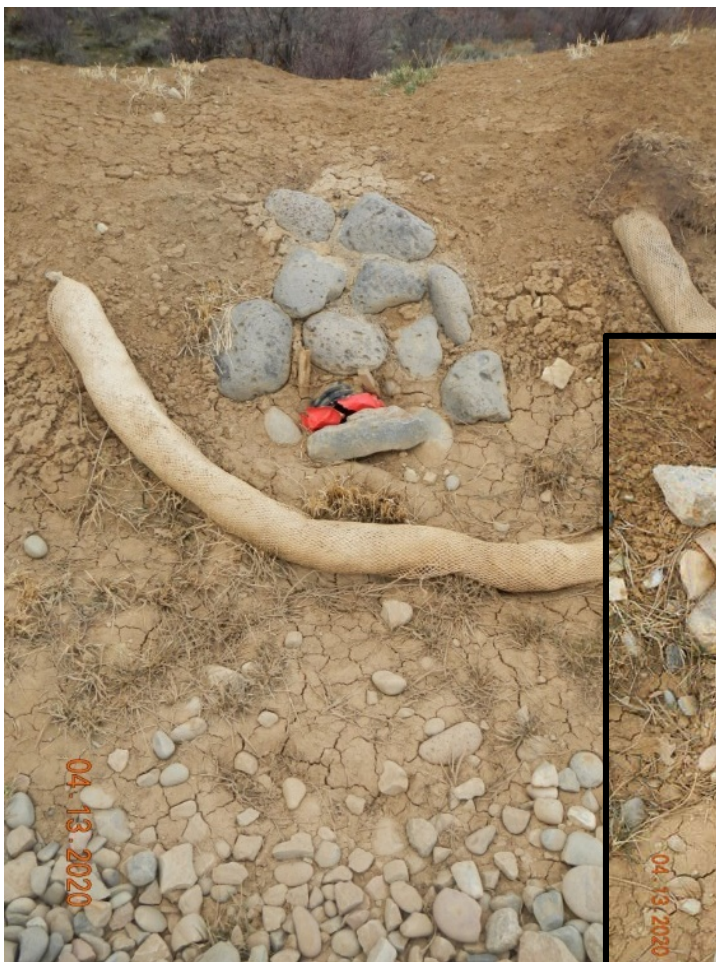
Photo#10: Blocked drains on Pad Fill slope edge.
