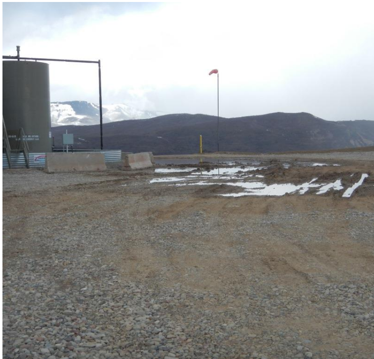
Photo#8: Ponding and degradation of pad surface.
