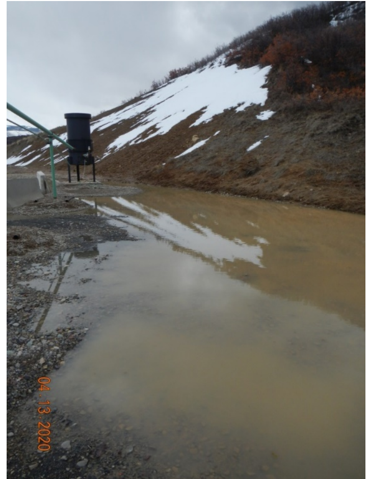
Photo#7: Ponding of stormwater.
