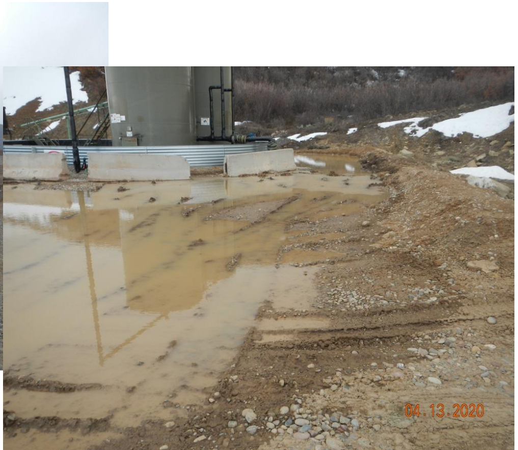
Photo#9: Ponding and degradation of pad surface
