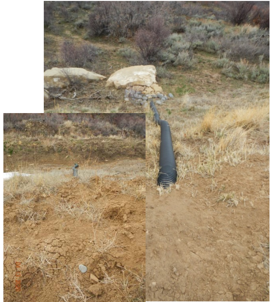
Photo#13: Flexible drains running to base of Fill slope.
