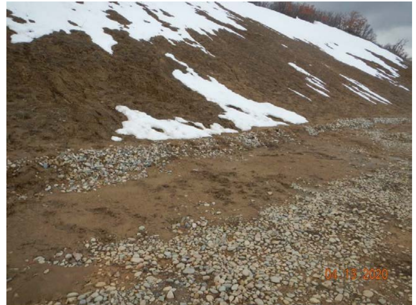
Photo#5: Erosion on Cut slope.
