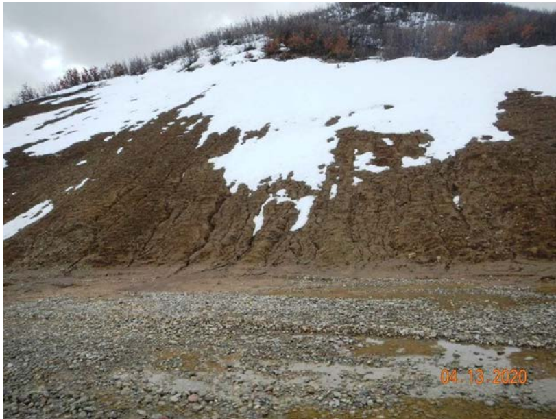
Photo#4: Erosion on Cut slope.
