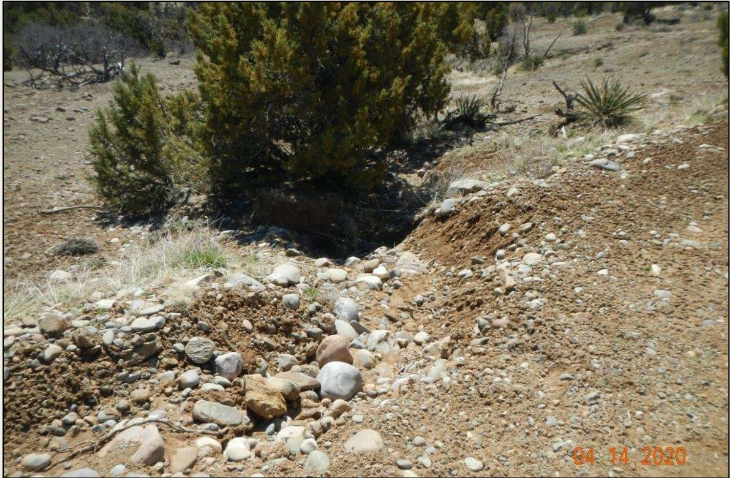
Photo 5. View of another erosional channel flowing off of the access road, that is not stabilized. Approximately 3-4 feet wide and deep.
