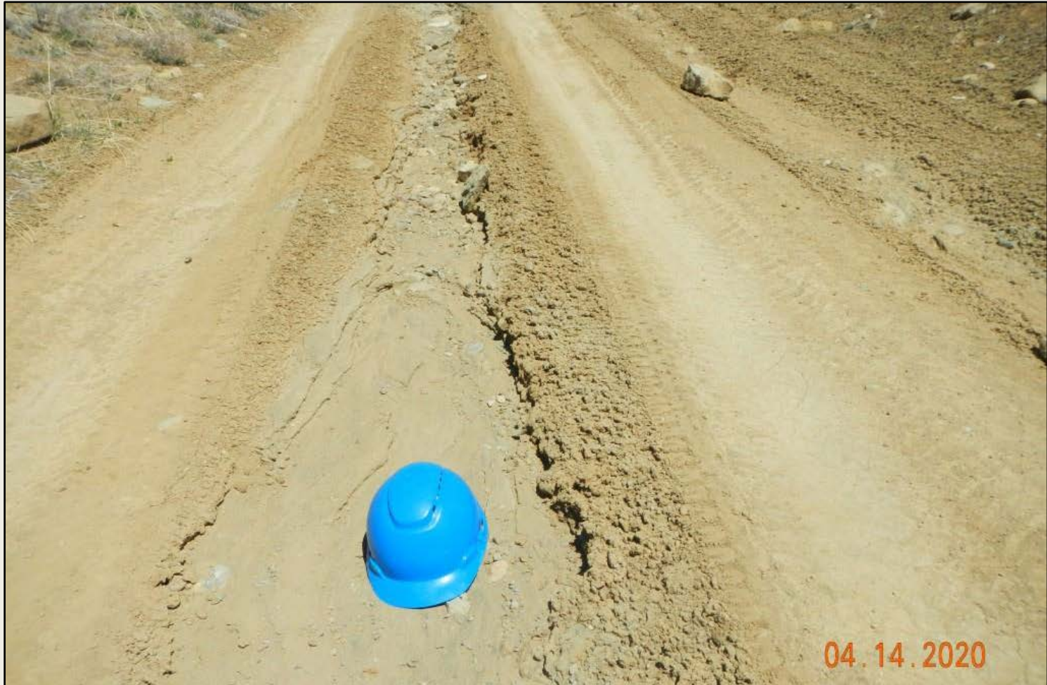
Photo 6. View of rutting and sedimentation on the access road, approximately 1.5 feet deep.
