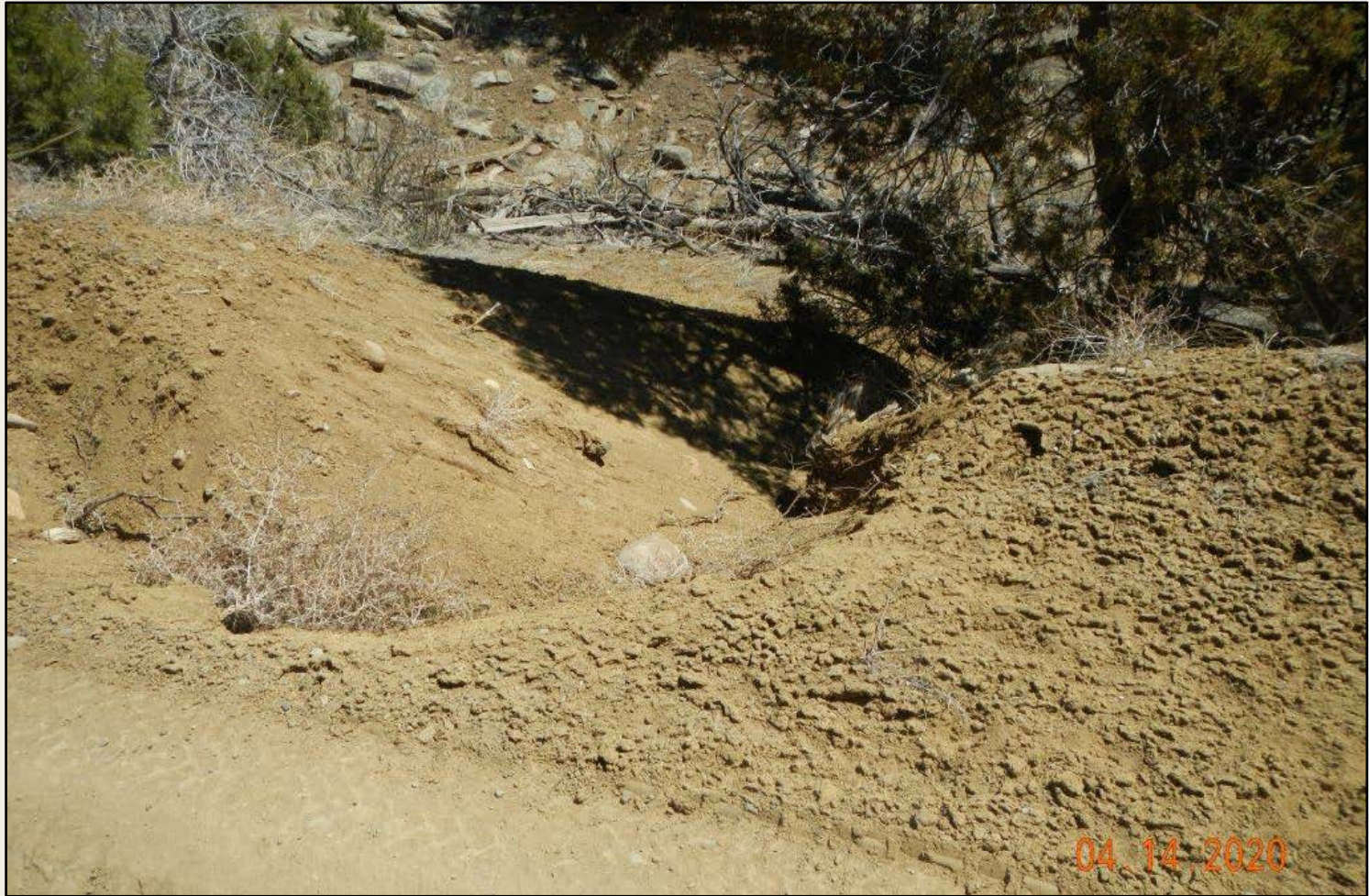
Photo 4. View of erosional channel flowing off of the access road, that is not stabilized. Approximately 2-3 feet wide, and deep.
