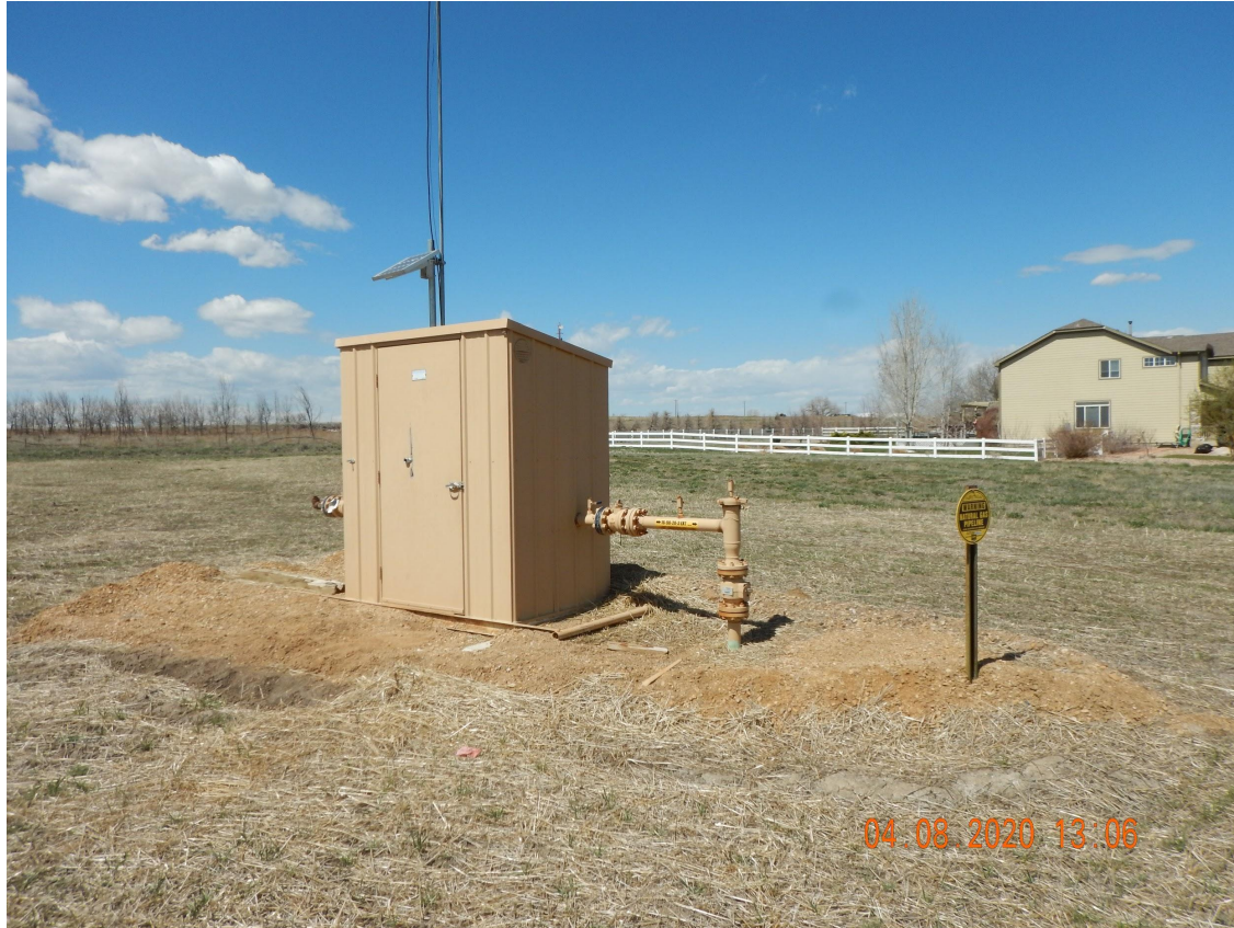
Photo 1. Photo taken from the well and battery location, facing Northwest. Photo illustrates Operator has failed to remove all equipment.
