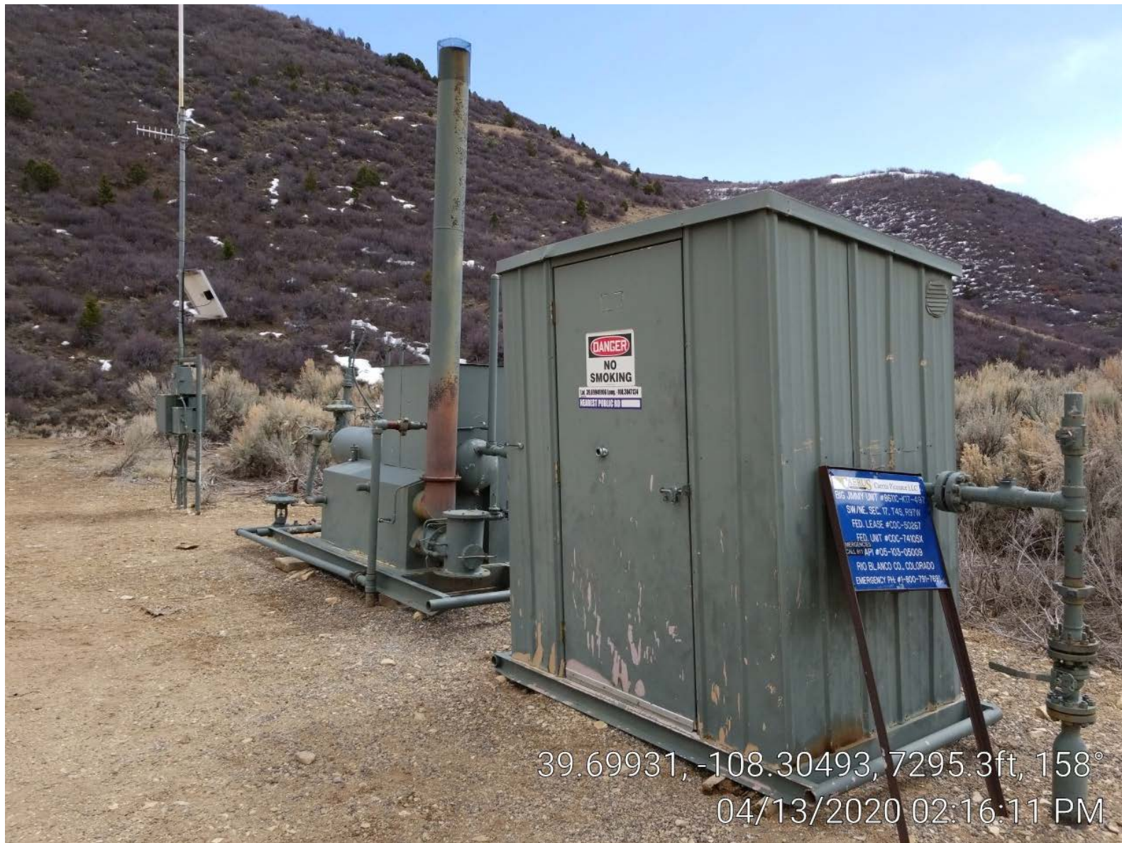
Photo 3. Meter building & separator.
