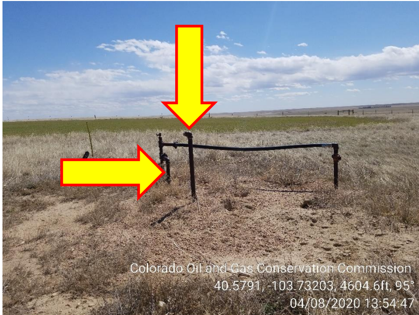
Photo 3 – Unmarked Risers
