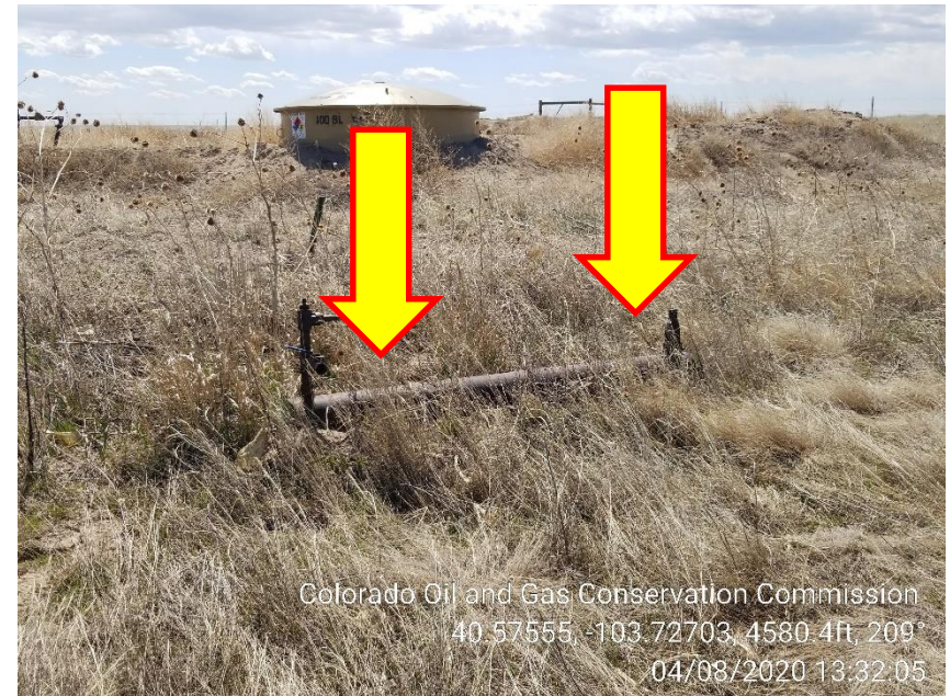
Photo 8 – Unused Volume Pot, west of Wellhead
