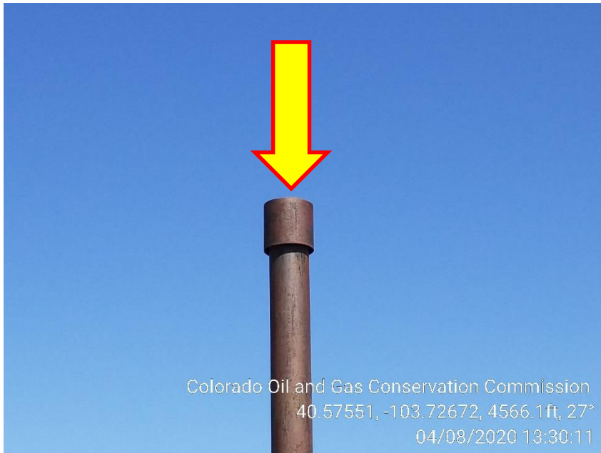
Photo 5 – Wildlife Screen missing from Separator
