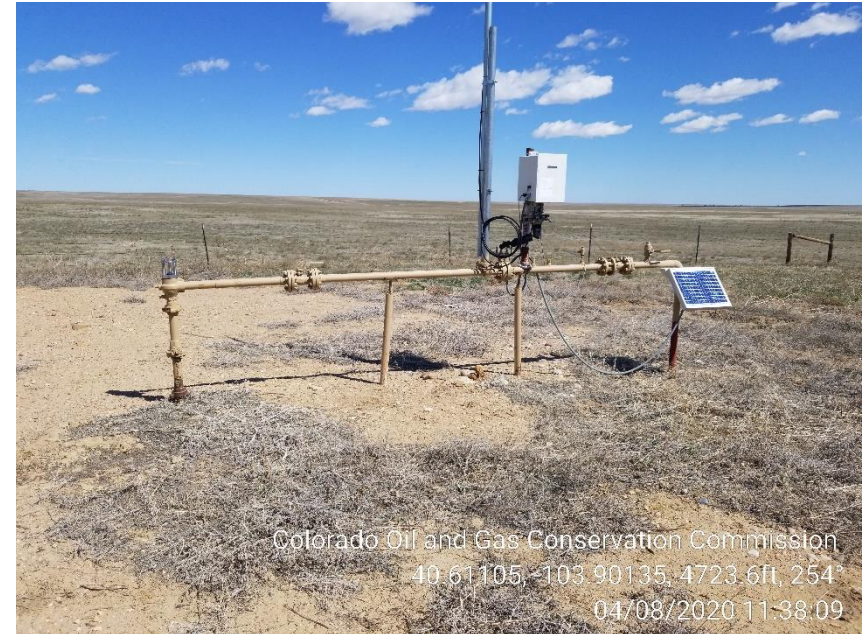
Photo 8 – Gas Meter on the Eastside of the Location
