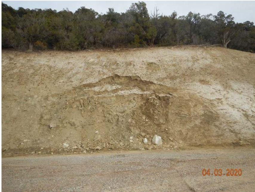
Photo#5: Slough on Cut slope.
