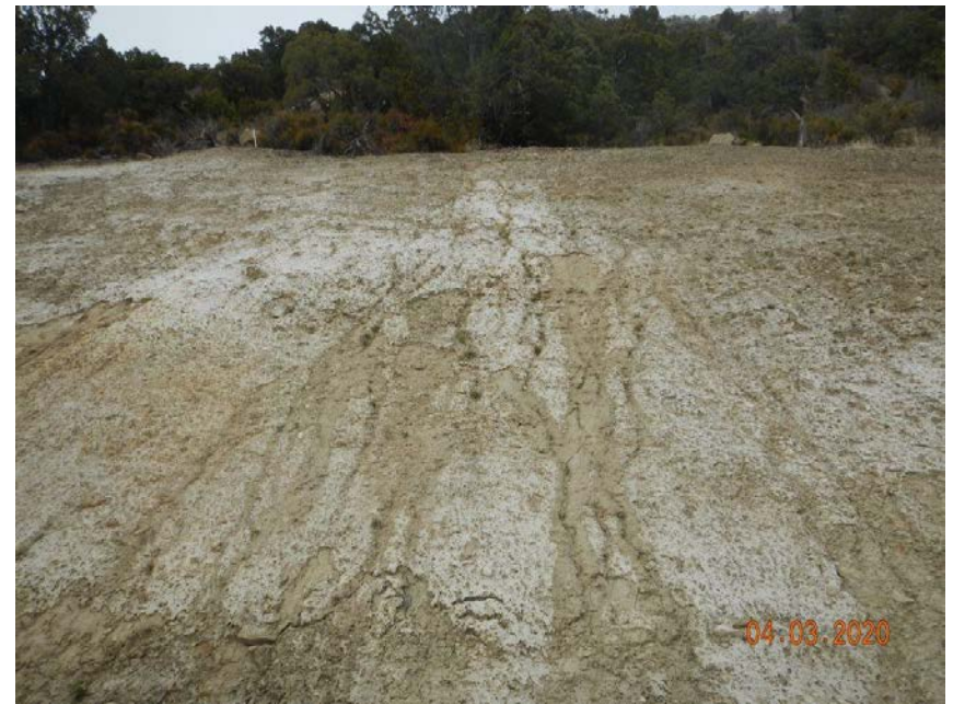
Photo#6: Erosion on Cut slope.
