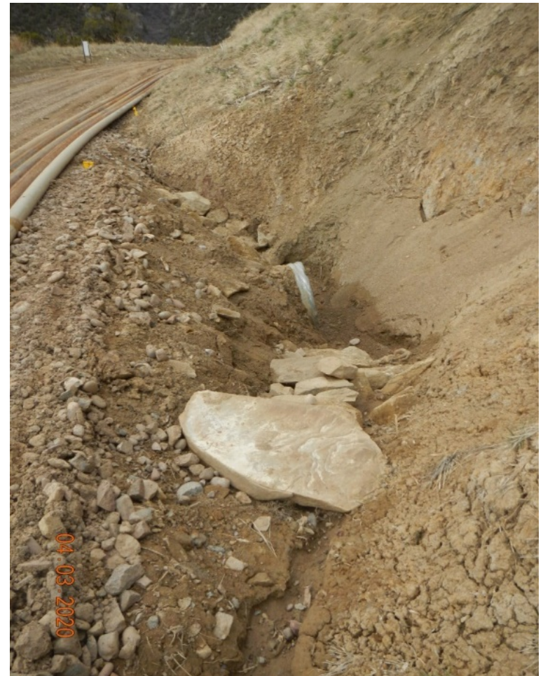
Photo#10: BMP at road culvert.
