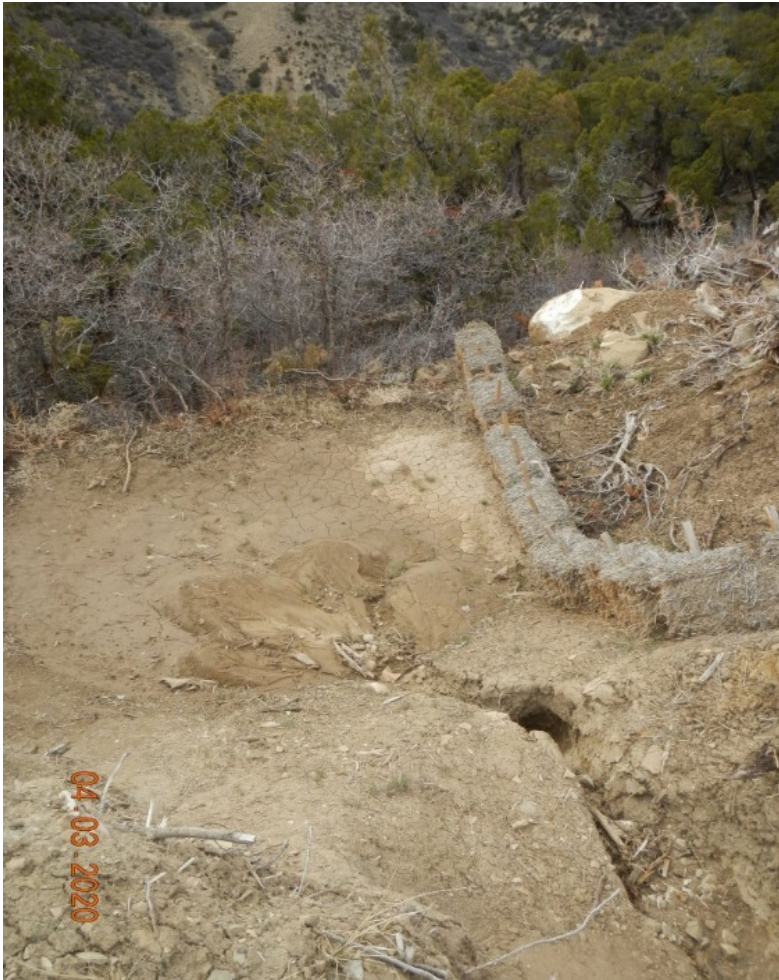
Photo#9: BMP at first drop to base of Fill.
