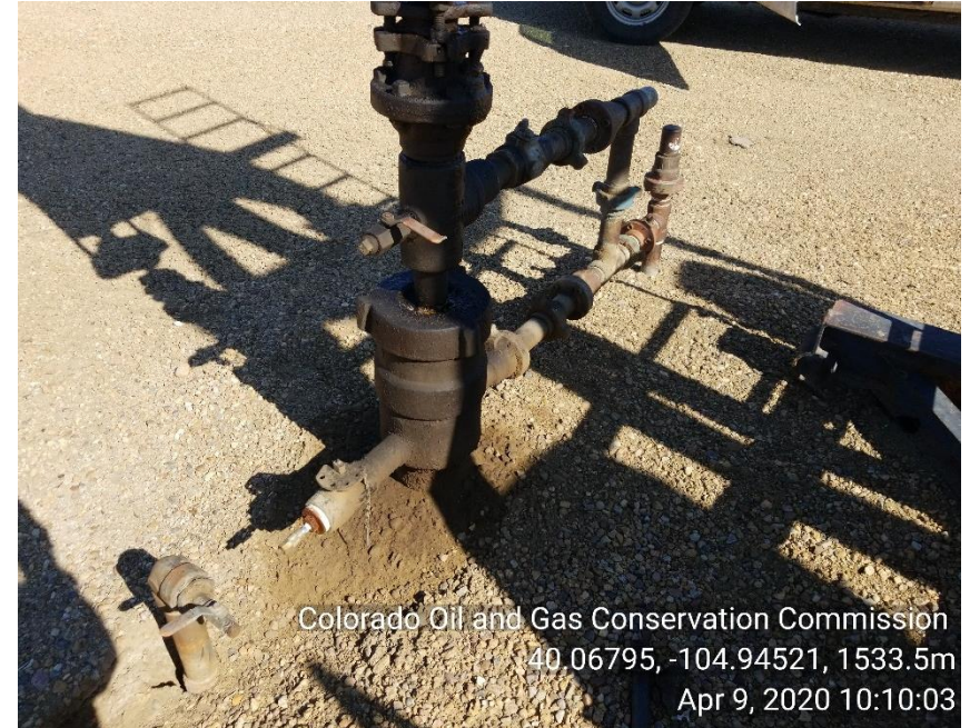
Photo 2 Stained soil around well head.
