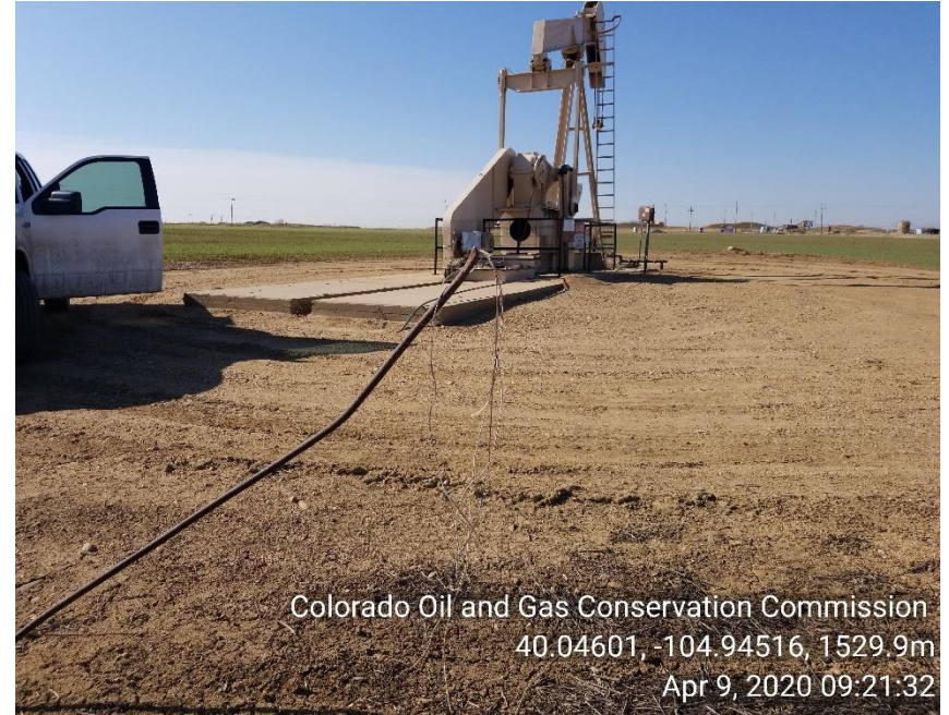
Photo 2 Electric pipe with exposed wires not marked not LOTO.
