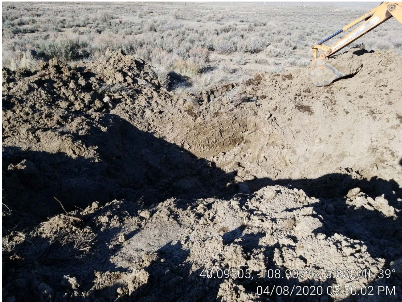
Photo 1. Hole dug at flow line leak.
