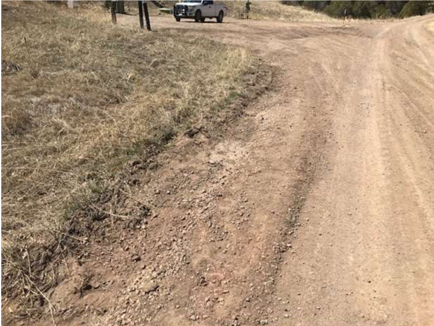
PHOTO 3: THE IMPACTED SOIL ALONG THE BAR DITCH WAS CLEANED UP.
