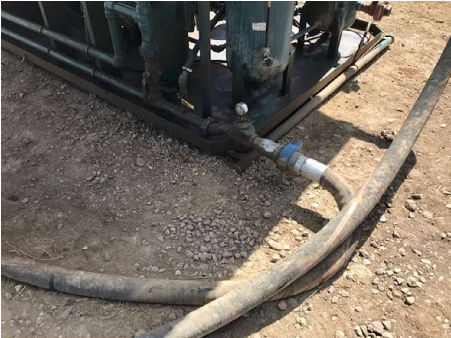
PHOTO 2: THE OIL ON THE LIQUID RING SKID AND THE GROUND WAS CLEANED UP ON 03/25/20. REPAIRS TO THE LIQUID RING WERE COMPLETED ON 04/08/20.
