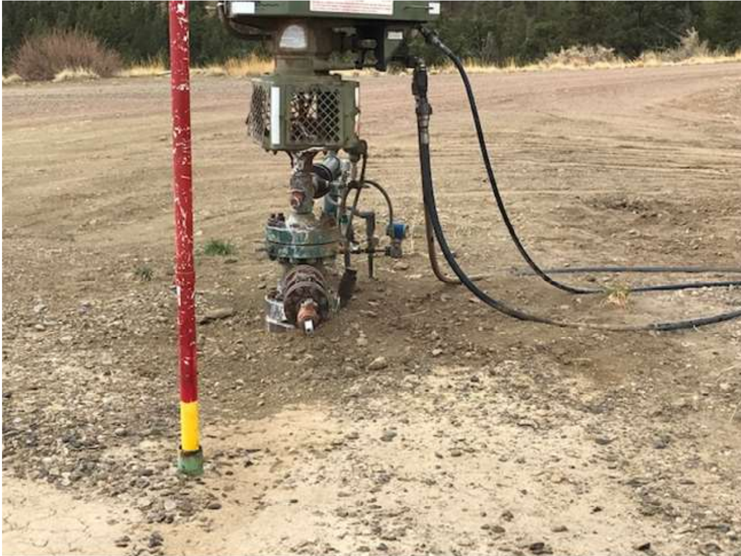
PHOTO 1: THE PACKINGS ON THE WELL HEAD WERE REPLACED TO ELIMINATE THE WATER LEAK. THE SOIL UNDER THE WELL HEAD WAS CLEANED UP.
