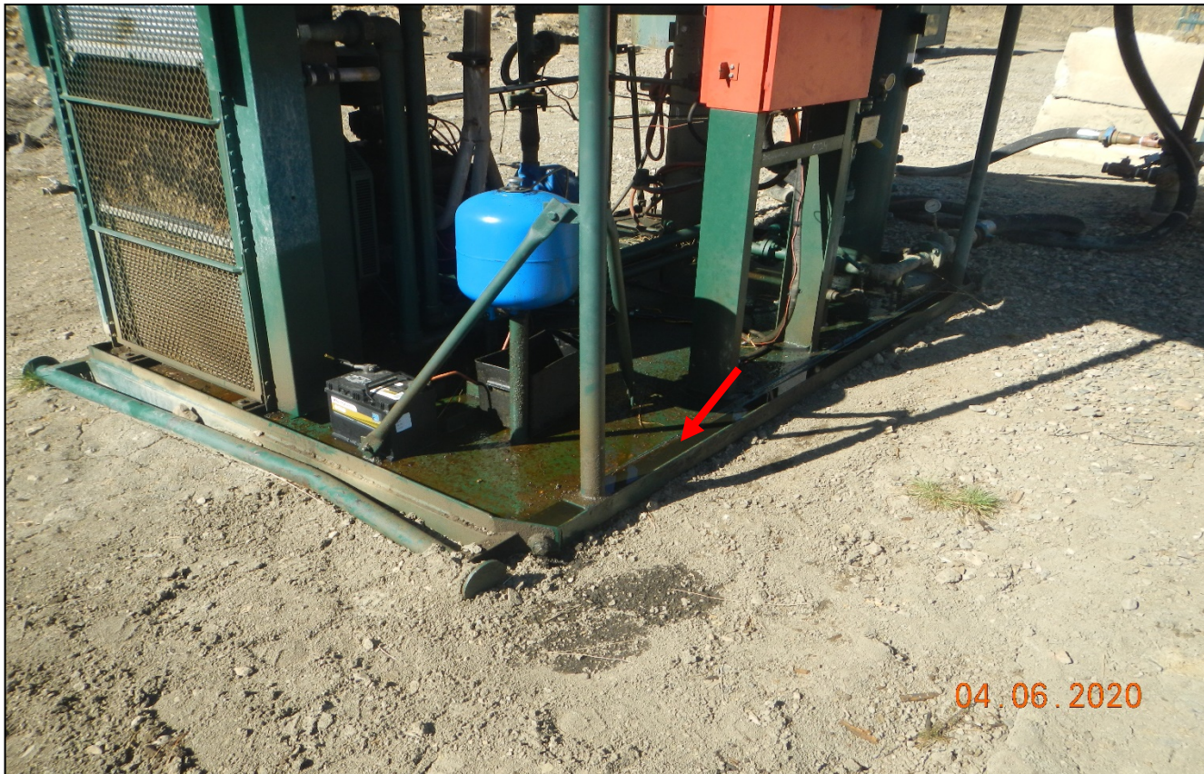
Photo 3. There is oil on the engine skid that will need to be cleaned up.
