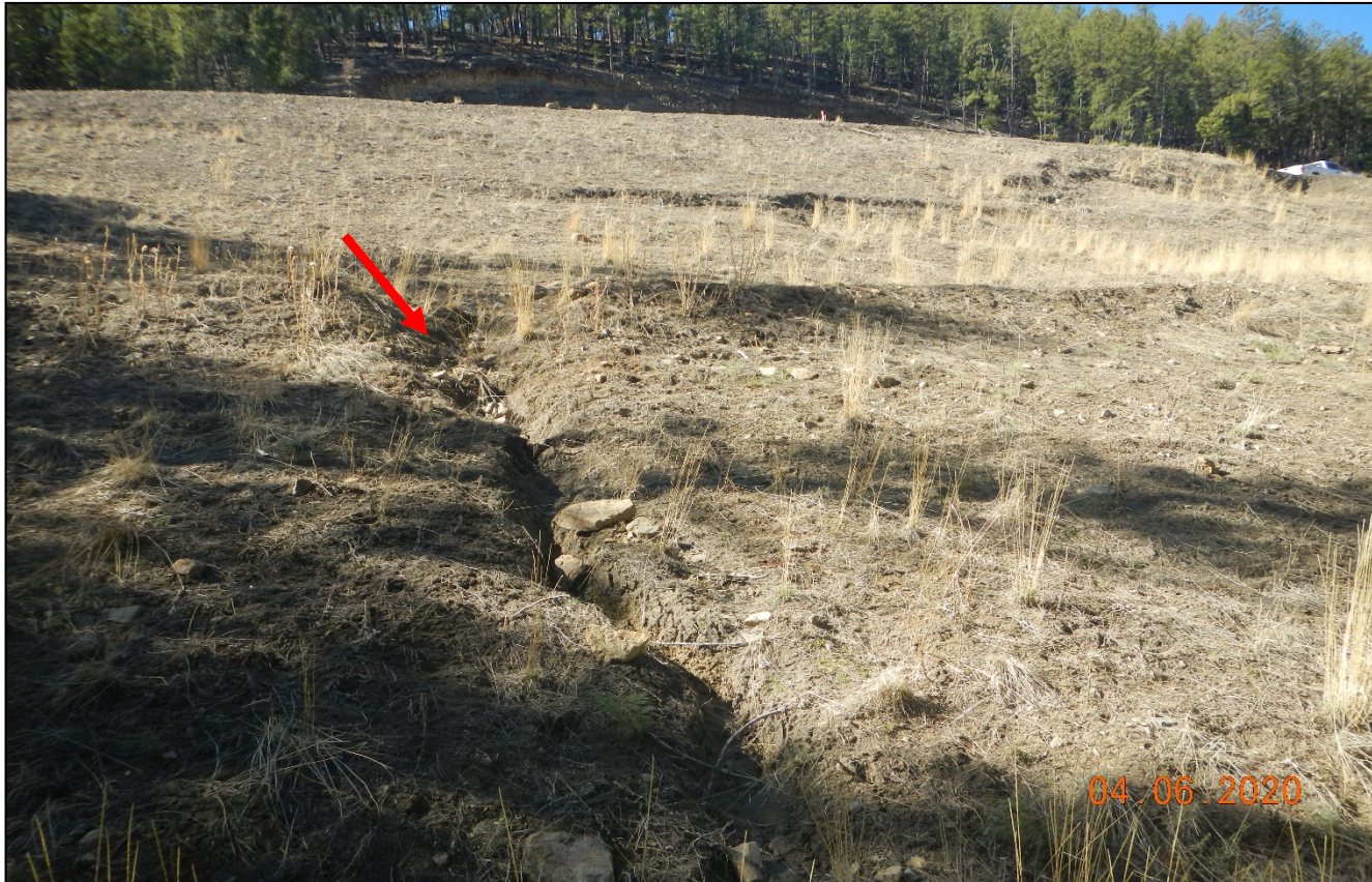
Photo 5. Facing southwest toward the fill slope. There is an erosion channel that has developed in this area.
