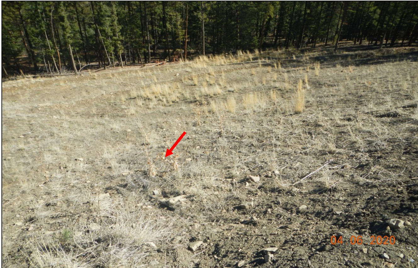
Photo 4. Facing down toward the fill slope. There were numerous noxious weeds observed along the fill slope during previous inspection which remain. (Canada thistle, Bull thistle. Noxious weed control will need to be performed in upcoming growing season.
