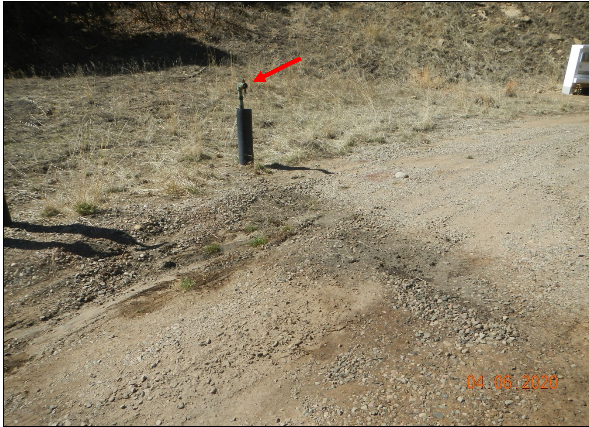
Photo 3. There is stained soils which appear to have been leaked out of pipe riser at SE side of location.
