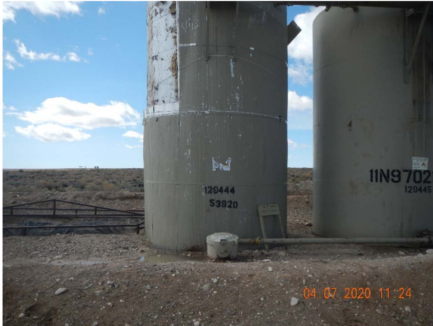
Photo 3. Label peeling off on left tank. Pit in tank battery behind left tank.
