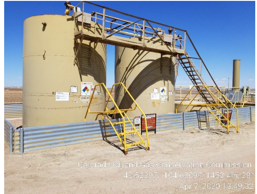
Photo 4: Tank Battery
