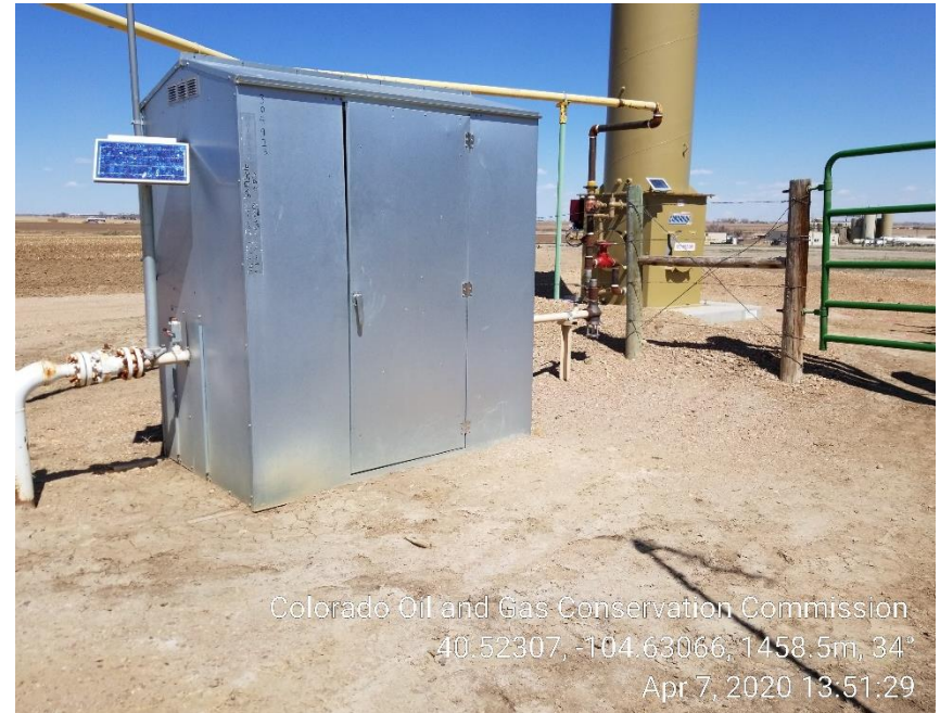
Photo 6: Disconnected gas meter
