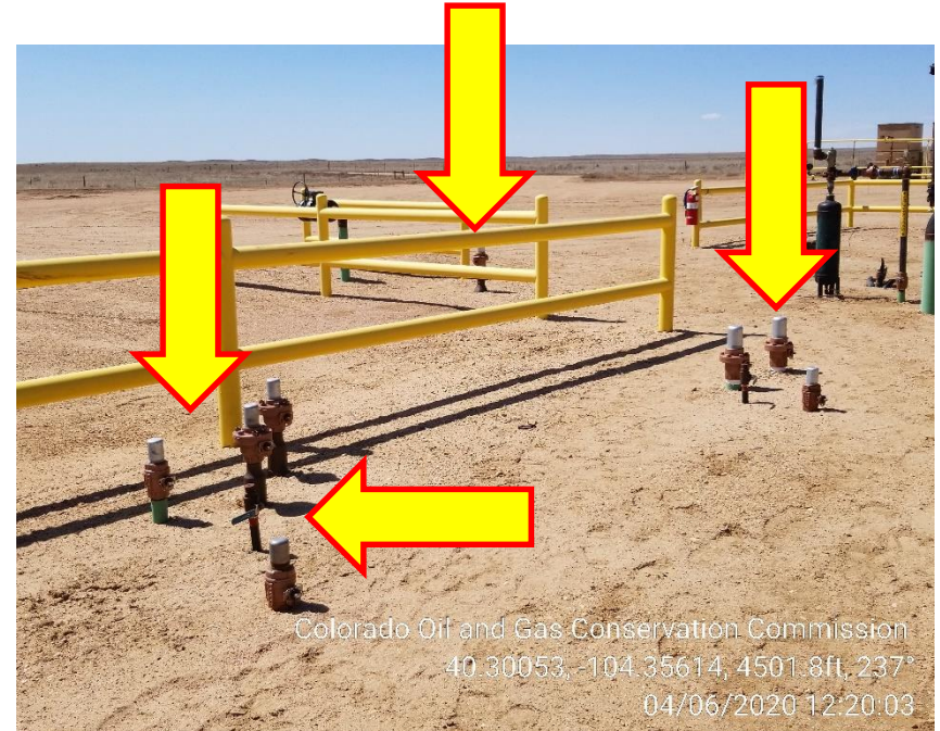
Photo 2 – Unmarked Risers south of the Separators
